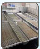
The flocculated suspended particles and chemical settle out in the sedimentation basin. Inclined plate settlers speed up the settling process. The sludge that is formed is pumped to the solids handling processes.
