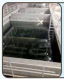
The treatment process starts with grit removal and addition of a flocculant. This combines with suspended particles to form "floc". It is mixed at progressively slower speeds.
