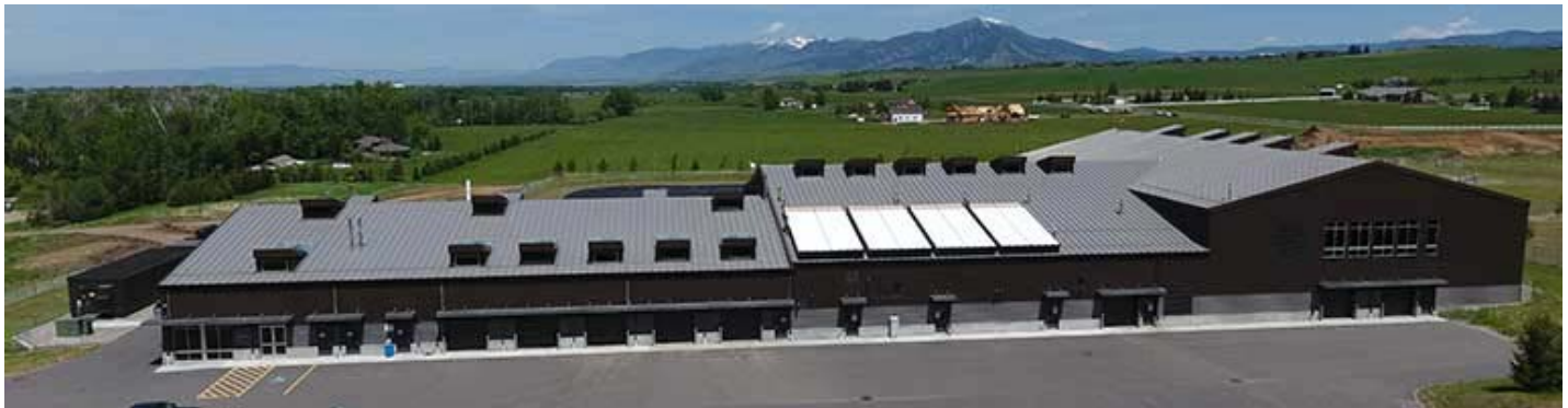
Figure 9. City of Bozeman Water Treatment Plant
