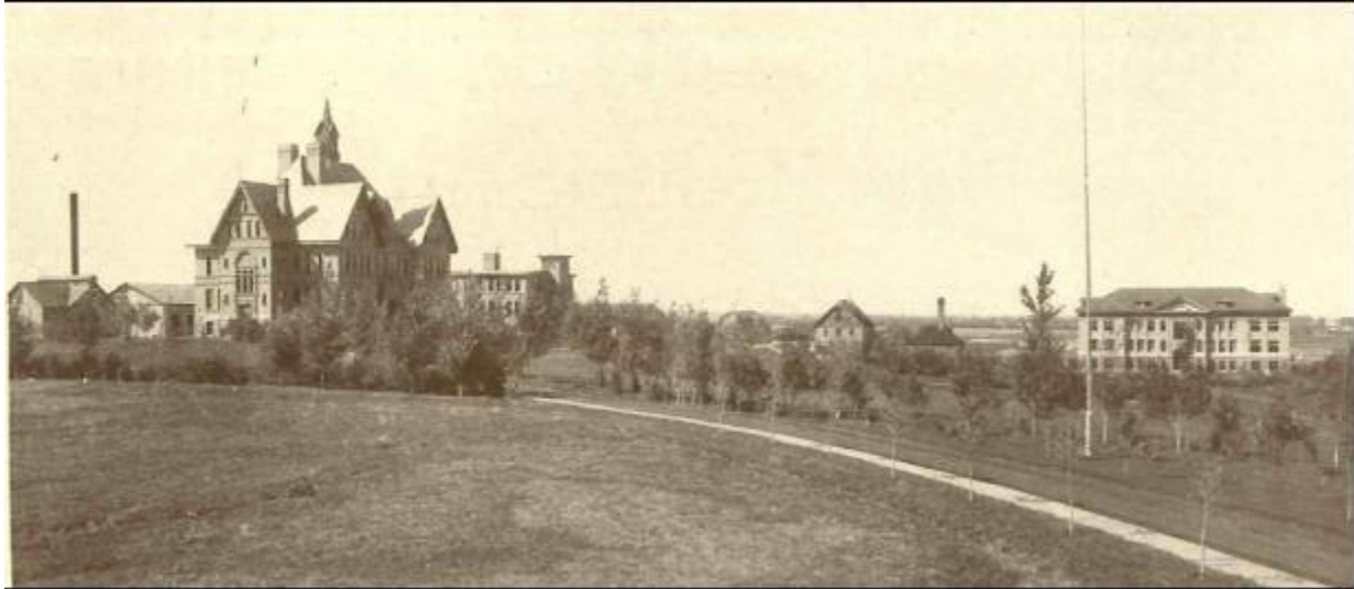
MSU Campus looking southwest, c. 1911. (From Left to Right: Mathematics Building, Heating Plant (background), Montana Hall, Chemistry Building, Taylor Hall, Heating Plant, Linfield Hall)
