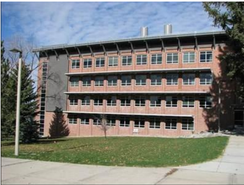
Photo 51 of 55. Cooley Laboratories (North Façade), 11/03/2012, Aspect: NW
