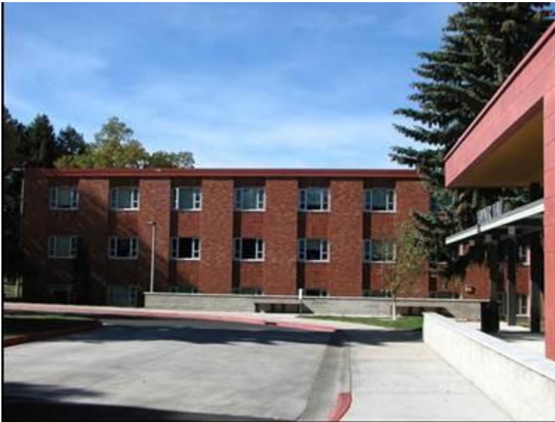
Photo 37 of 55. East Elevation of Hapner Hall's West Wing with new entrance on south façade in foreground, 10/07/2012, Aspect: W
