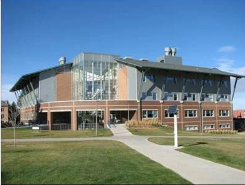
Photo 48 of 55. Chemistry and Biochemistry Building (Southeast Façade), 11/03/2013, Aspect: NW
