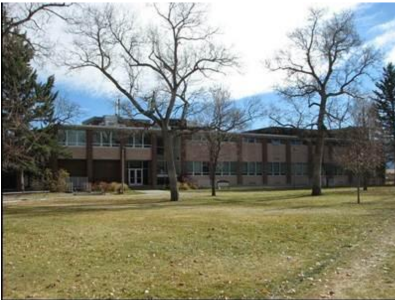
Photo 33 of 55. A.J.M. Johnson Hall (West Façade), 11/03/2012, Aspect: SE
