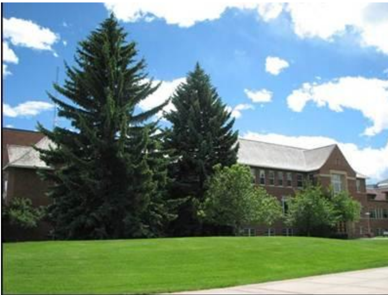
Photo 13 of 55. Strand Student Union from Centennial Mall, 06/20/2013, Aspect: SW
