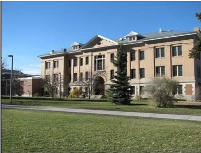
Photo 19 of 55. Linfield Hall (East Façade), 11/03/2012, Aspect: SW
