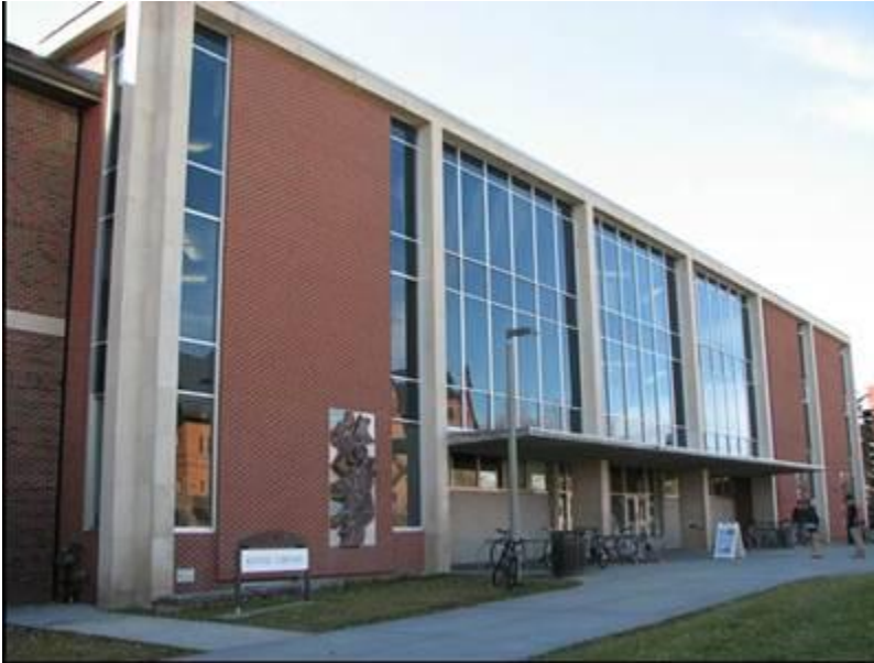
Photo 38 of 55. 1960 Renne Library Addition (North Façade), 11/03/2012, Aspect: SW
