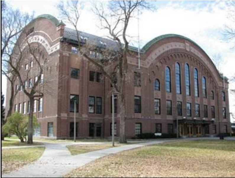
Photo 26 of 55. Romney Gymnasium (North Façade and East Elevation), 11/03/2012, Aspect: SW
