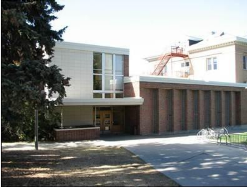
Photo 32 of 55. 1953 Addition to Linfield Hall (Linfield South, East Façade), 10/06/2012, Aspect: NW
