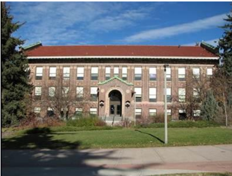
Photo 25 of 55. Lewis Hall (South Façade), 11/03/2012, Aspect: N
