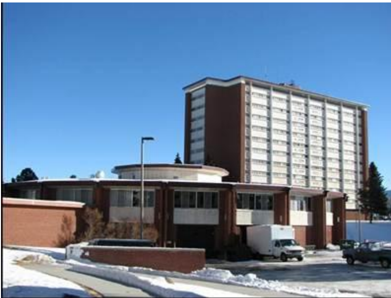
Photo 39 of 55. Hedges Complex (West Elevation of Food Service Building and South Hedges), 01/05/2013, Aspect: SE
