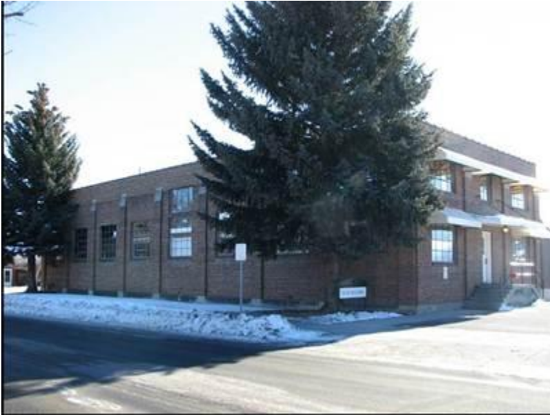
Photo 30 of 55. Plew Building (West Façade and North Elevation), 01/05/2013, Aspect: SE
