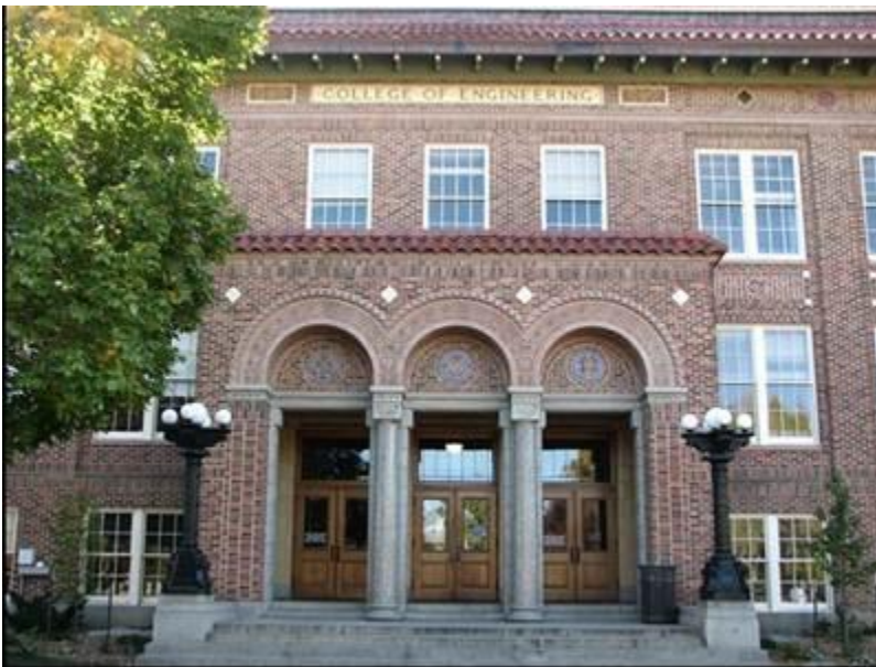
Photo 21 of 55. Roberts Hall Entrance (North Façade), 10/07/2012, Aspect: S
