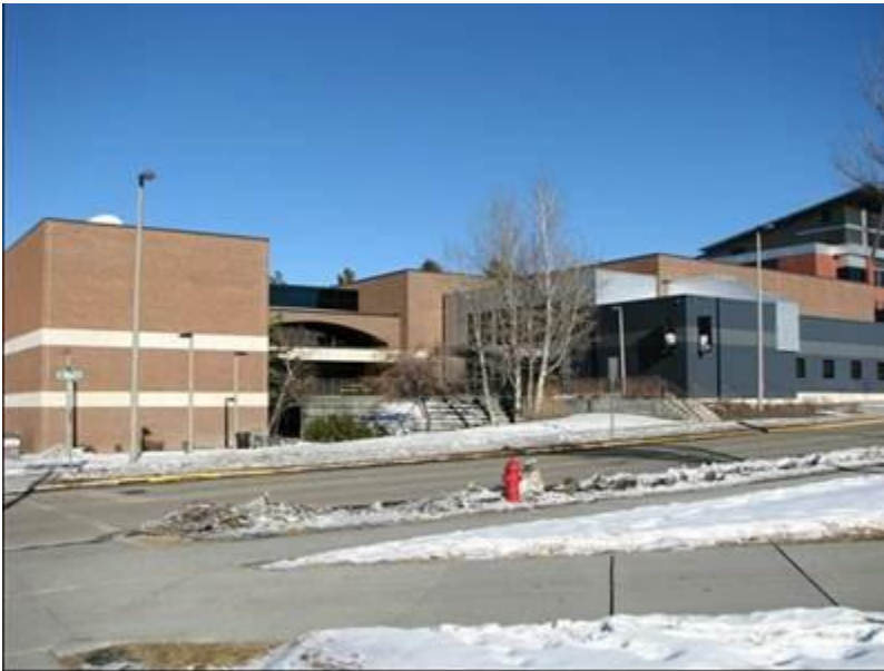
Photo 45 of 55. Visual Communications Building and Black Box Theater Addition (South Façade), 01/05/2012, Aspect: NE
