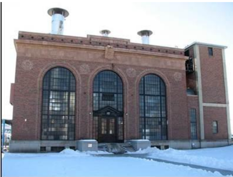
Photo 23 of 55. Heating Plant (North Façade), 01/05/2013, Aspect: S
