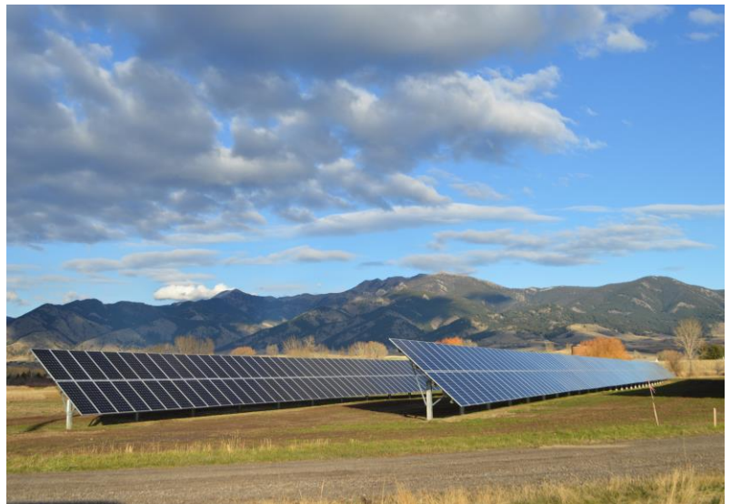
Bozeman Solar Project Pilot, NorthWestern Energy’s 385kW solar PV array at the City of Bozeman Water Reclamation Facility. Photo: Orion Thornton
