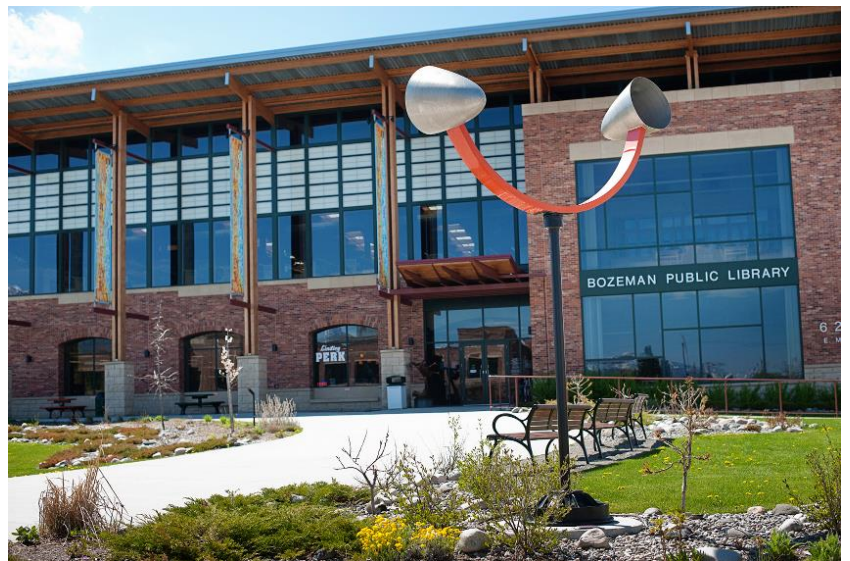
Bozeman Public Library is LEED Silver Certified and is equipped with a 16.7kW solar PV array.
