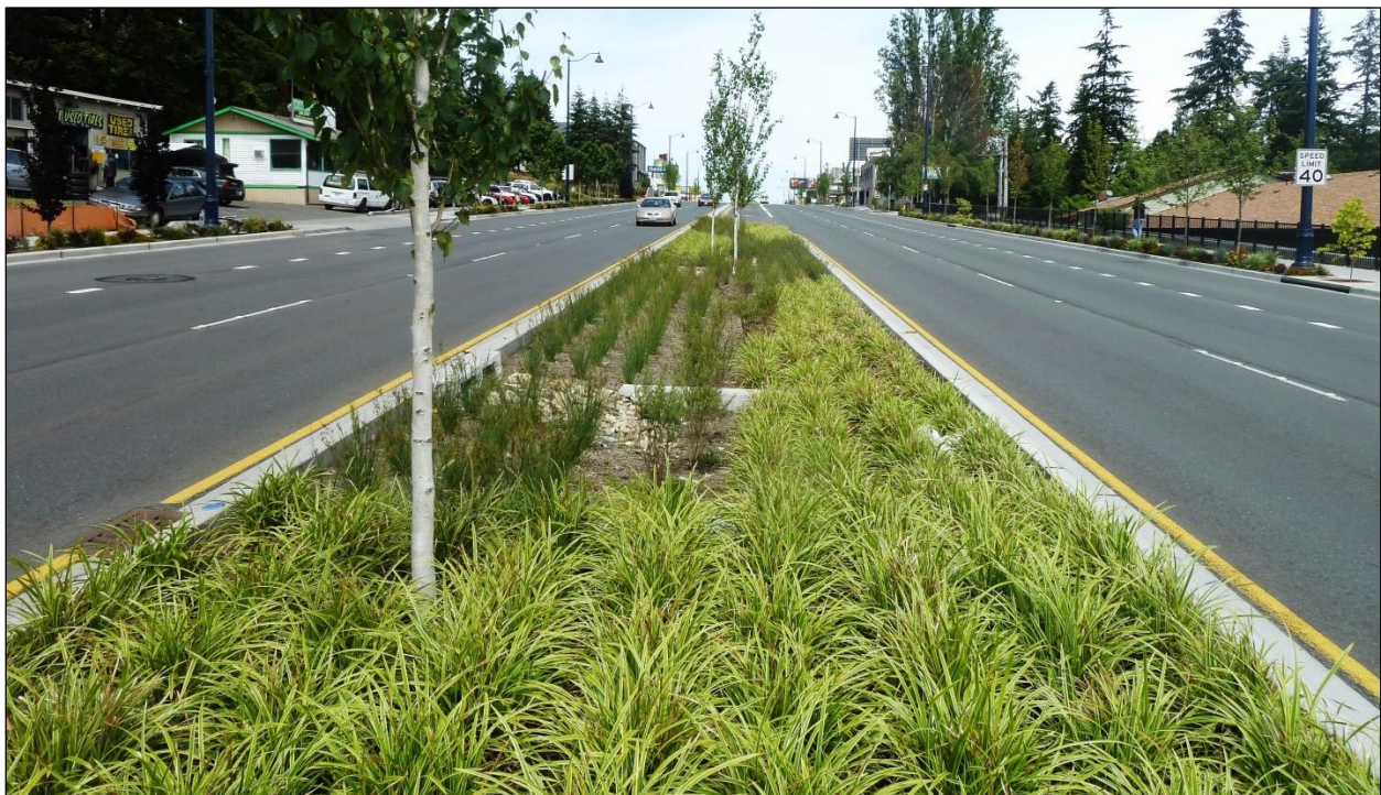
Figure 5.3-3. Bioretention Area within Roadway Median
