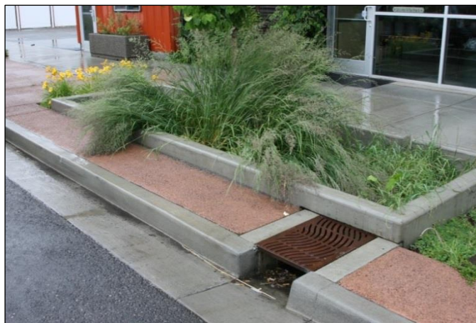
Figure 5.3-6. Offline Bioretention Area
