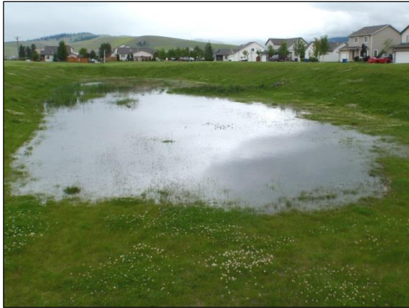
Figure 5.2-1. Infiltration Basin Source: HDR
