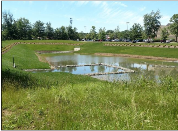
Figure 5.8-1. Wet Detention Basin Source: HDR
