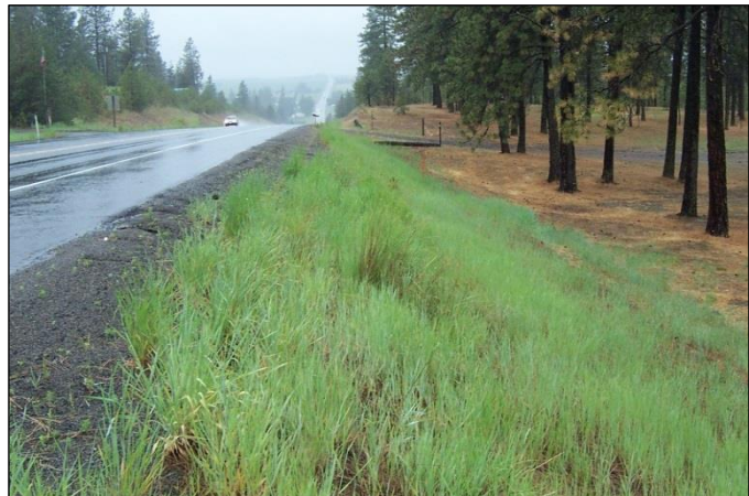
Figure 5.5-2. Dispersion Area Adjacent to a Roadway
