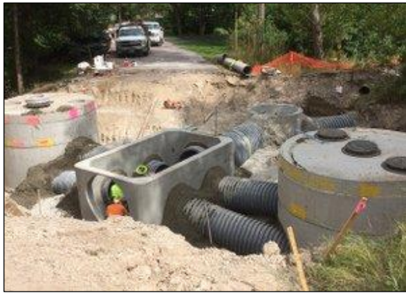
Figure 5.9-1. Proprietary Treatment Device Installation
