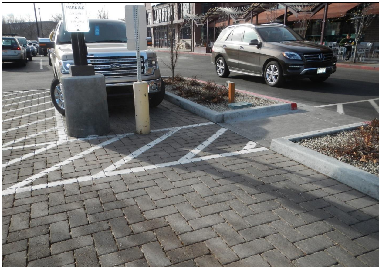
Figure 5.4-2. PICP Parking Lot Application
