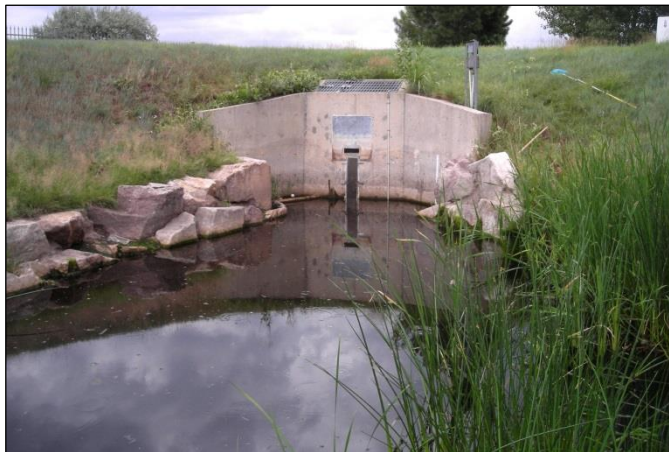
Figure 5.7-4. Micropool and Outlet Structure
