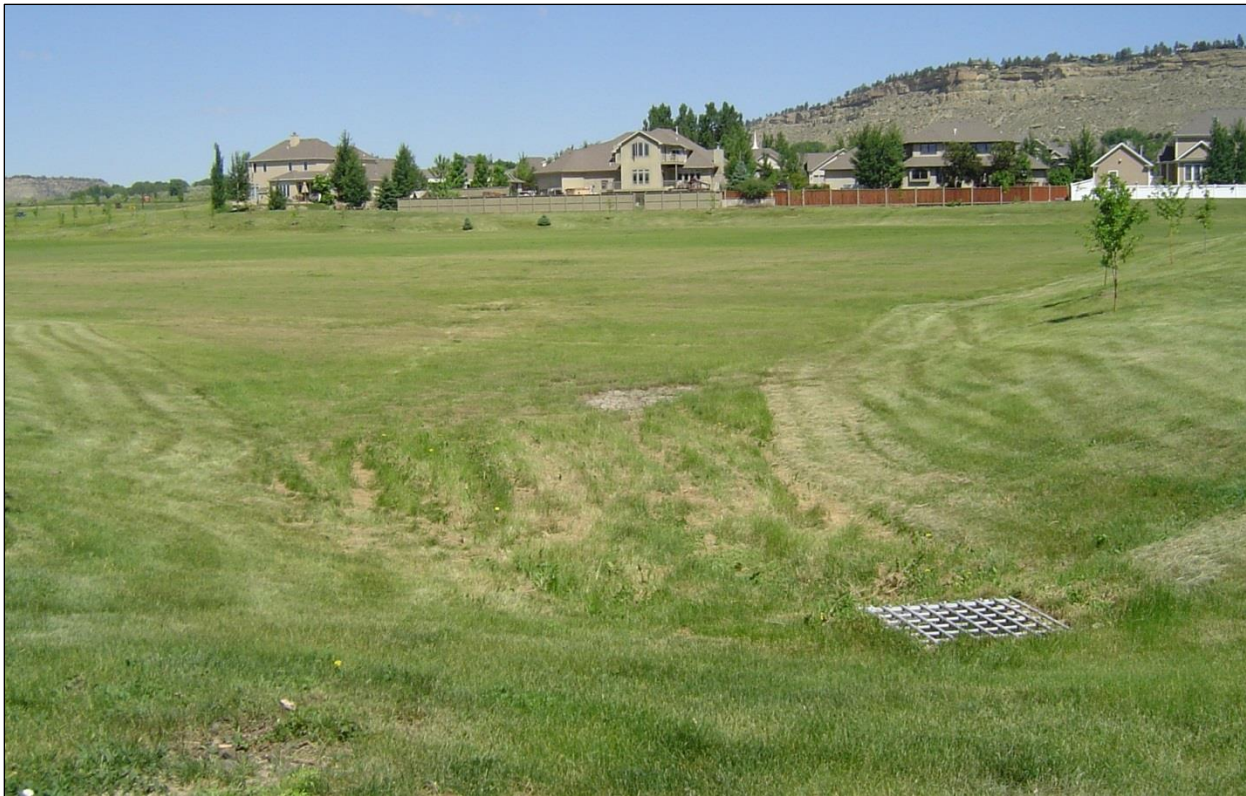
Figure 5.7-2. Detention Basin in Billings, Montana
