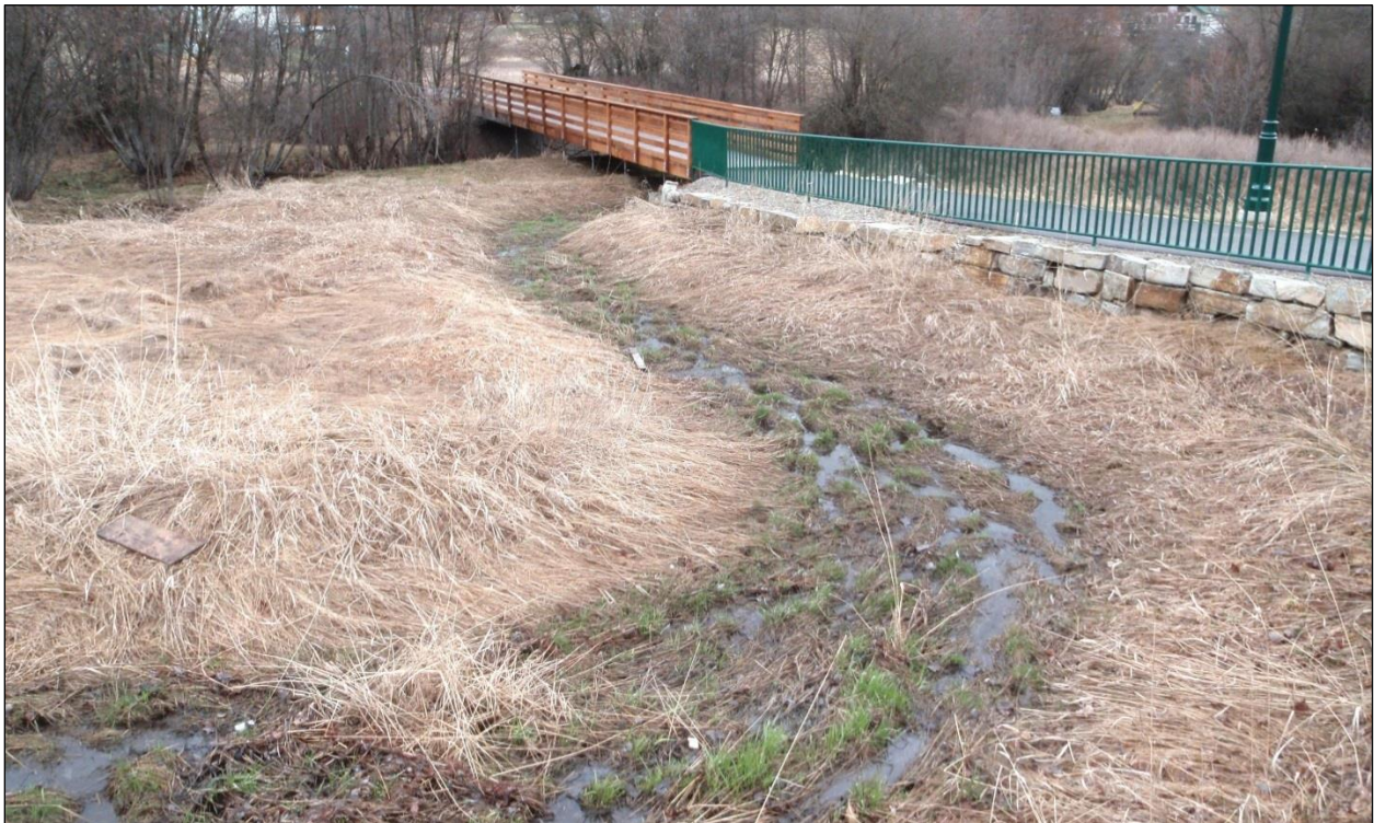
Figure 5.6-2. Meandering Biofiltration Swale
