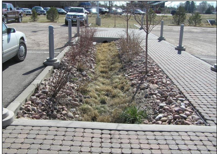
Figure 5.4-4. PICP and Bioretention System Treatment Train Source: Courtesy of Altitude Training Associates, LLC
