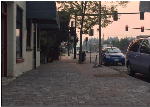
Figure 5.4-1. Permeable Interlocking Concrete Pavers in Bozeman
