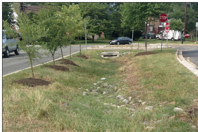
Figure 5.2-2. Infiltration Basin with Outlet Structure Source: HDR
