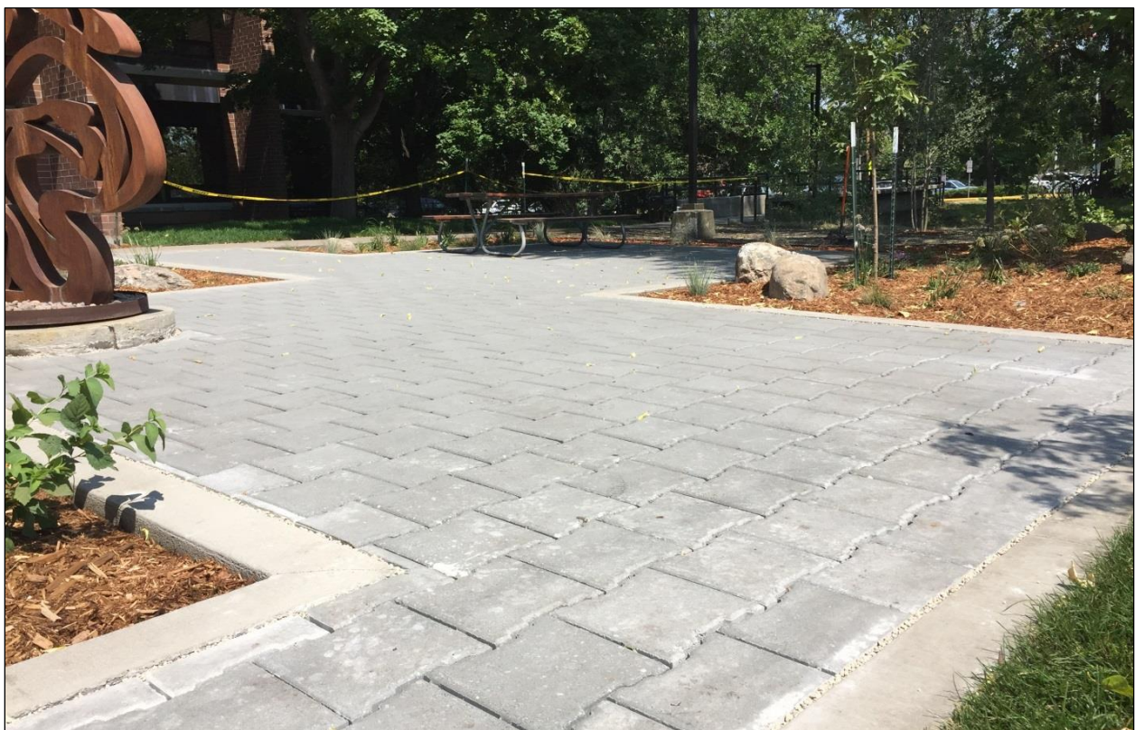
Figure 2-5. Permeable Interlocking Concrete Pavers Walkway Application
