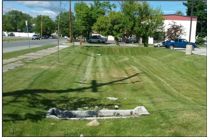
Figure 5.6-4. Level Spreader
