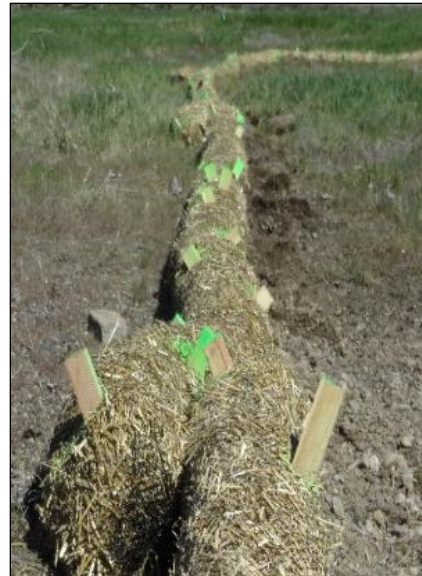
Image 12 - Properly installed straw wattle.
