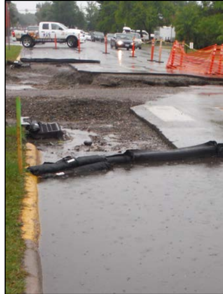
Image 15 - Properly installed weighted wattle.
