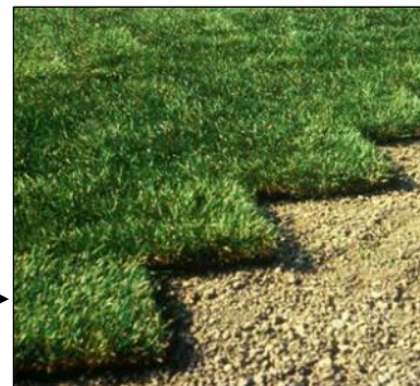
Stabilize Disturbed Area Sod →
