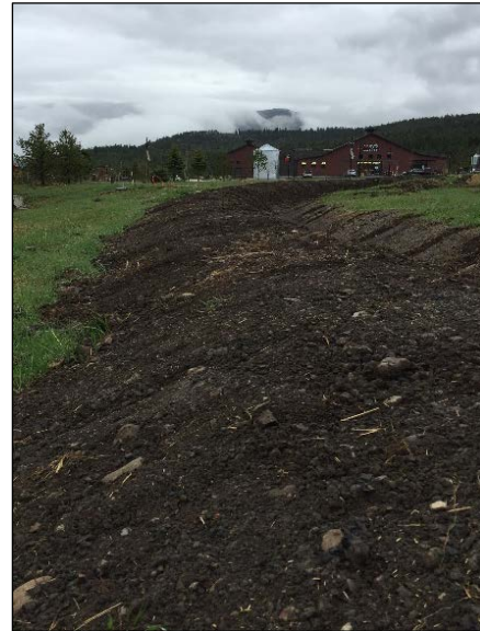
Image 19 - Installed compacted earthen berm
