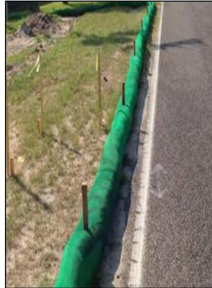
Image 13 - Properly installed filter sock. Image from filtrex.com
