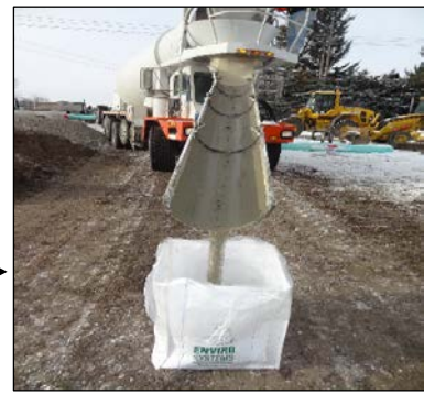
Control Concrete Waste Washout Bag →
