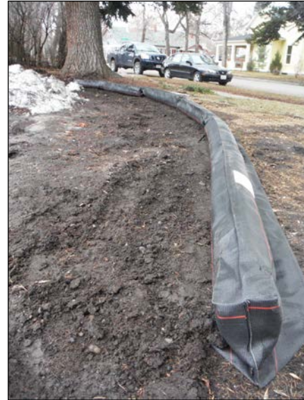
Image 9 - Properly installed foam wattle with apron
