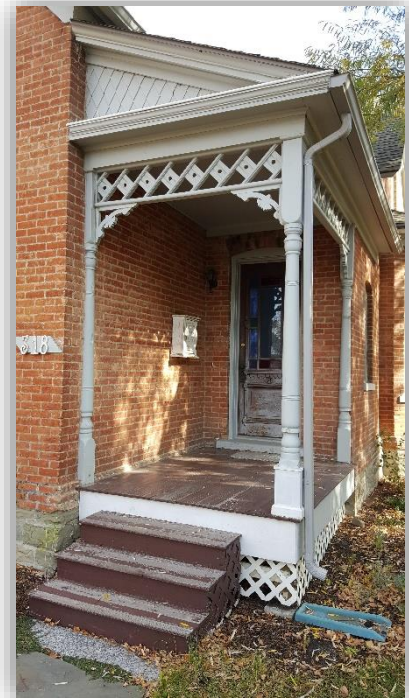
The intricate turned wood detailing represents a significant character defining feature on this remaining historic porch in the South Tracy Historic District.
