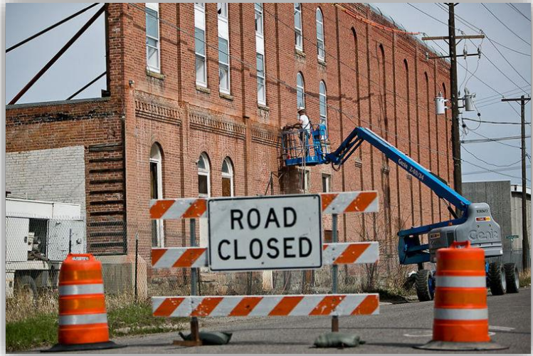
Source: Bozeman Daily Chronicle, “Demolition Begins on Lehrkind Brewery Wall,” April 21, 2014
