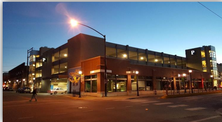
The new City parking garage provides a similar scale, massing and material pallet compatible with historic Main Street, yet contemporary in its building type and interpretation. Ground floor tenant space and the public transit hub reinforce pedestrian activity.
