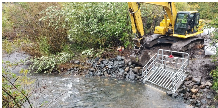
Image 19. Installation of Automated Diversion Structure
