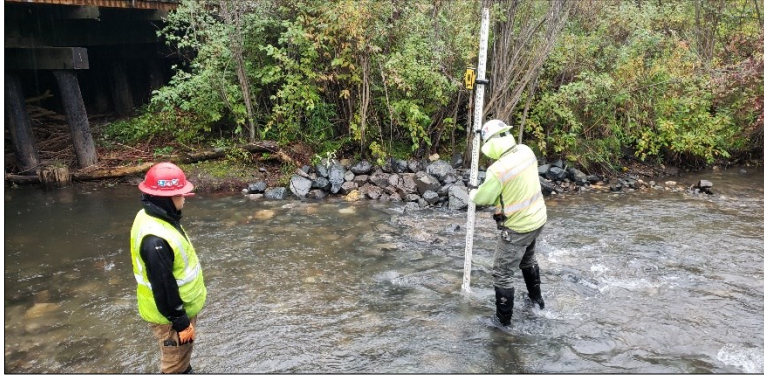
Image 20. Installation and Measurement of Aquatic Species Rock Ramp
