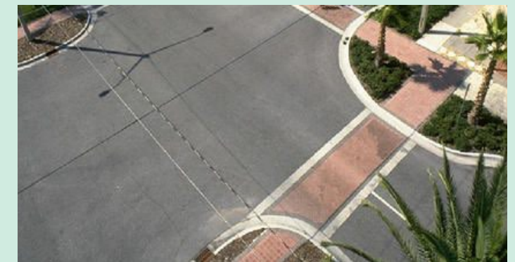
Figure 4.21 Curb bulb out
