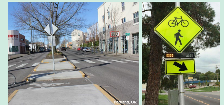
Figure 4.20 Median refuge island and RRFB
