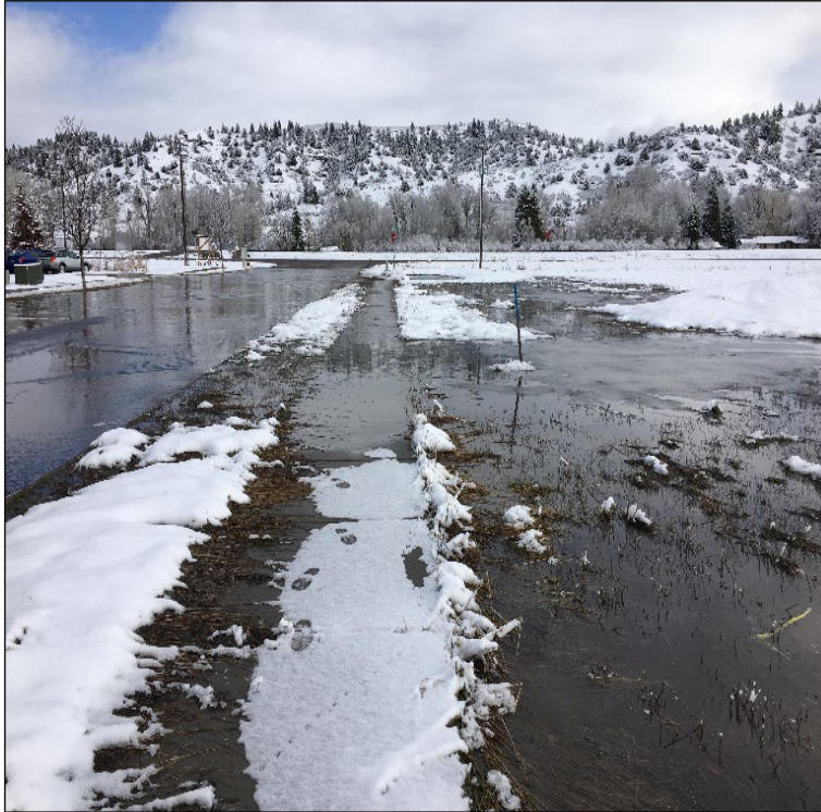
Graphic 1.0.1: Street flooding resulting from clogged infrastructure
