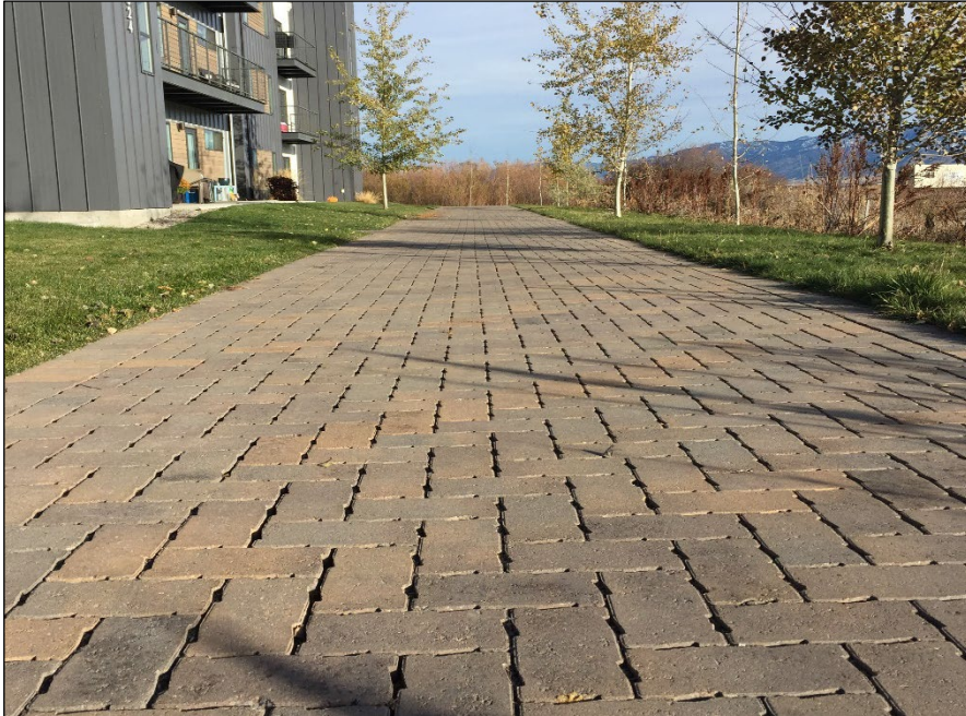
Graphic: 9.0.1: Permeable Paver Walkway
