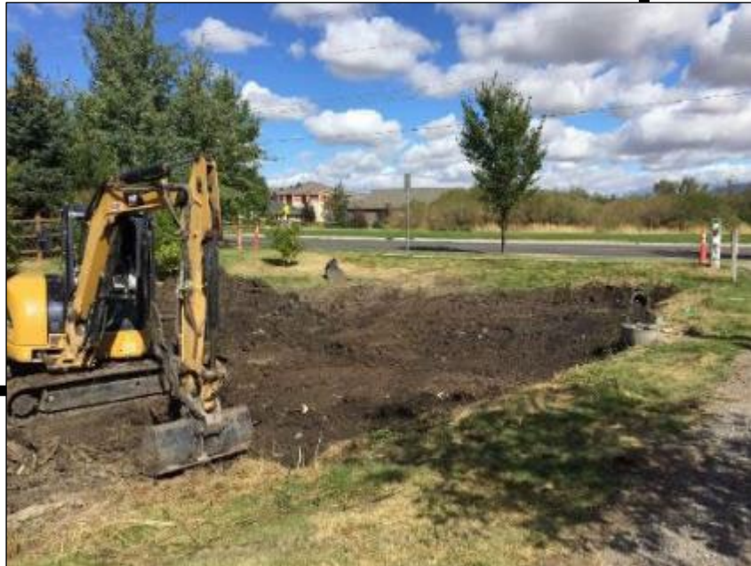
Image 6.0.2 Stormwater basin restoration
