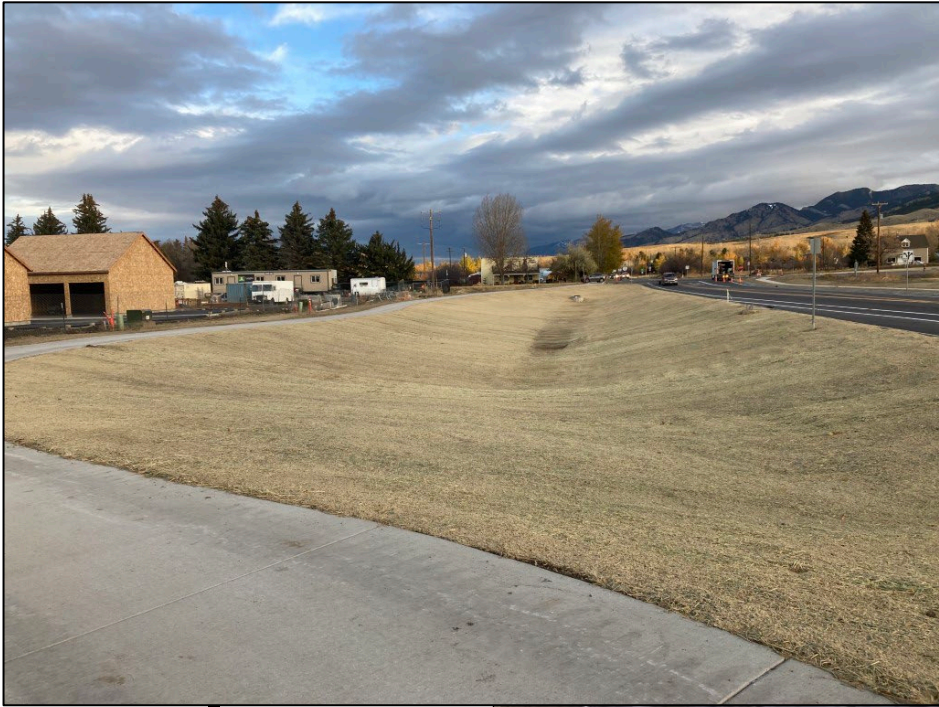
Graphic 5.0.1: Recently constructed and stabilized stormwater pond
