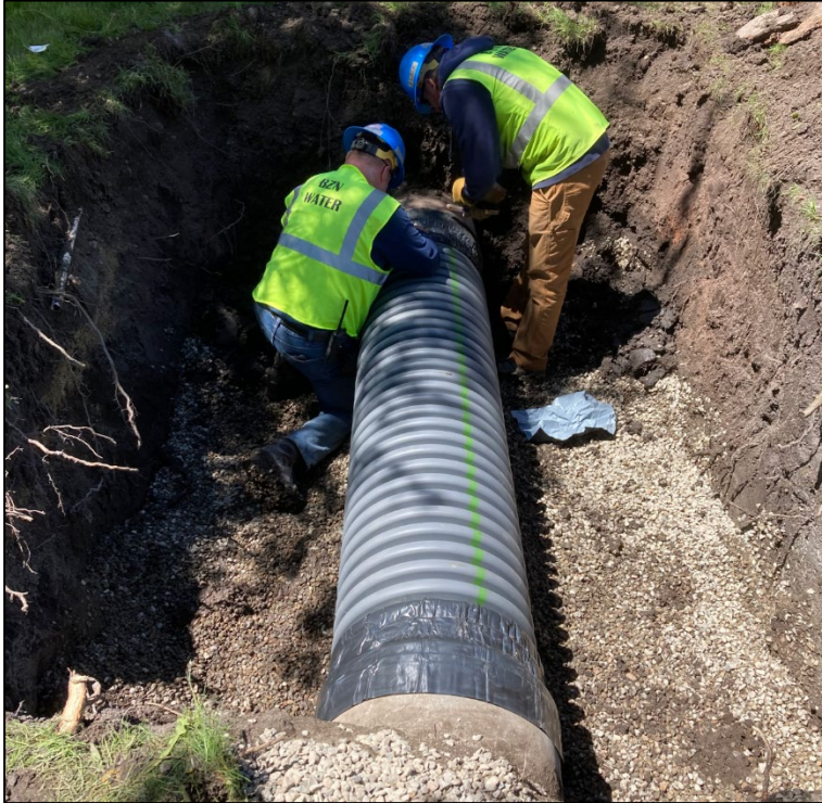
Graphic 2.0.1: Stormwater pipe replacement and repair
