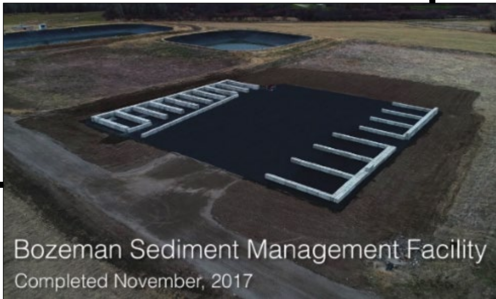
Graphic 7.0.2: Sediment management facility
