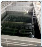
The treatment process starts with grit removal and addition of a flocculant. This combines with suspended particles to form "floc". It is mixed at progressively slower speeds.
