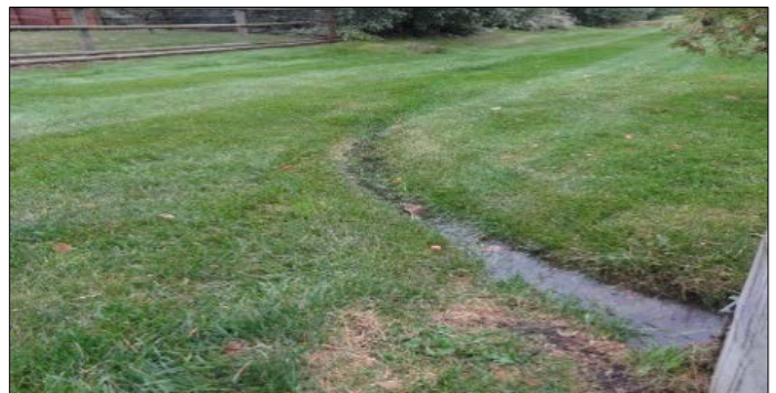
Image 3 - Erosion causing channelized flow
