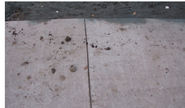
Concrete shared use path with saw cut joints in Billings, MT
