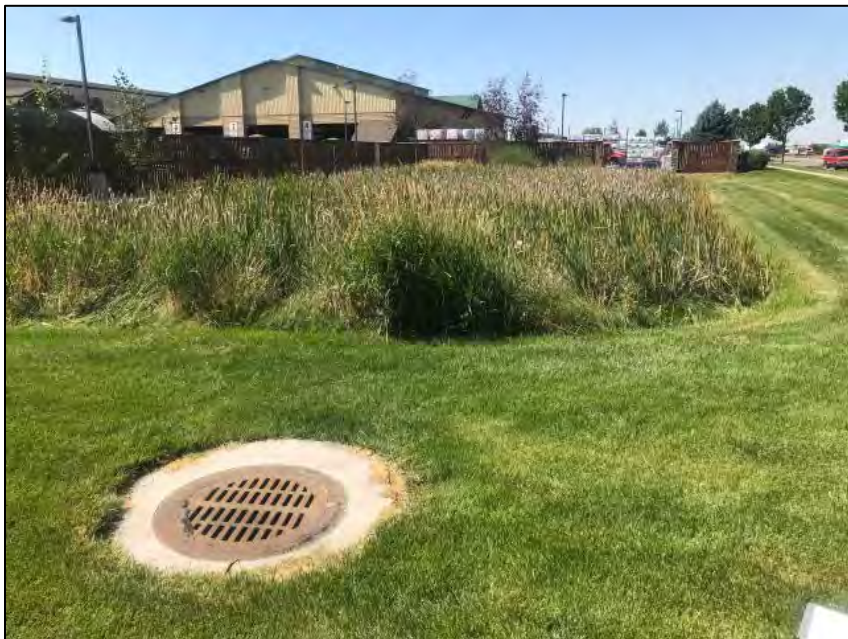
Image 1 Facility overview (west view).
