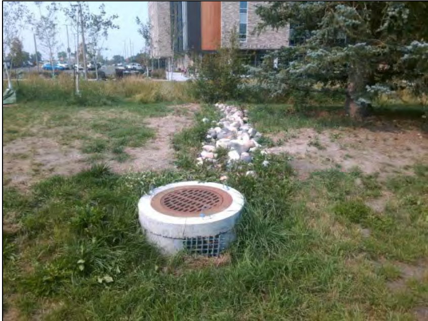
Image 3 Outlet structure. Overflow is cobble stone to background (west view).
