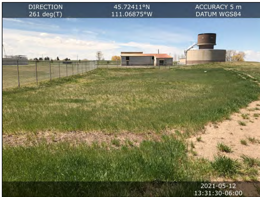
Image 1 Facility overview, evidence of mowing since last inspection. (west view)
