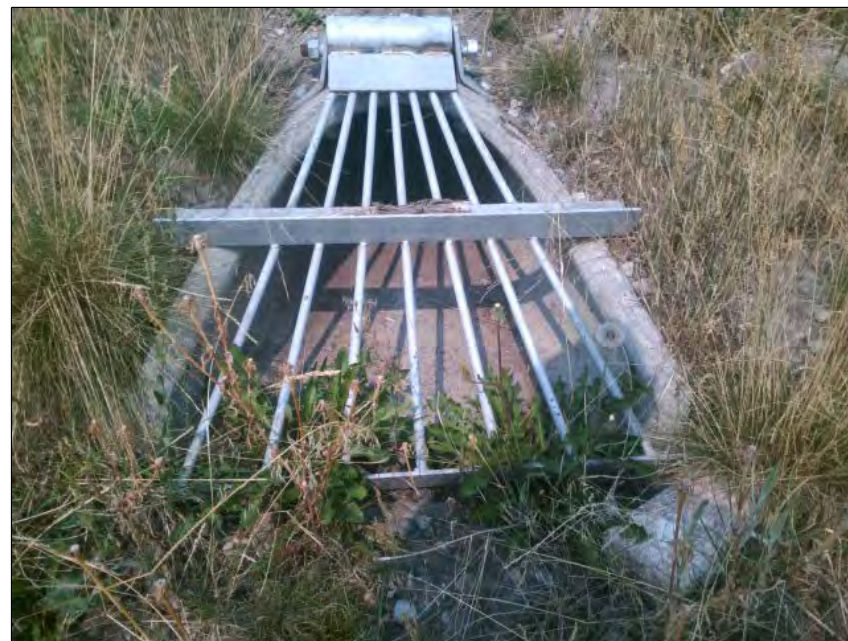
Image 2 Outlet structure (northwest view).
