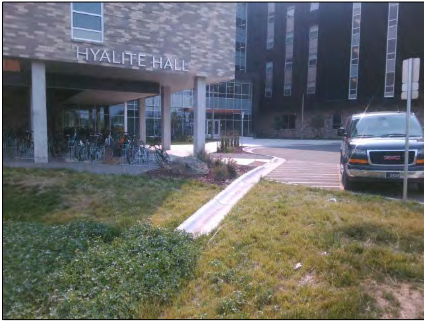
Image 3 Inlet 2; concrete curb and gutter from Hyalite Hall front parking lot.
