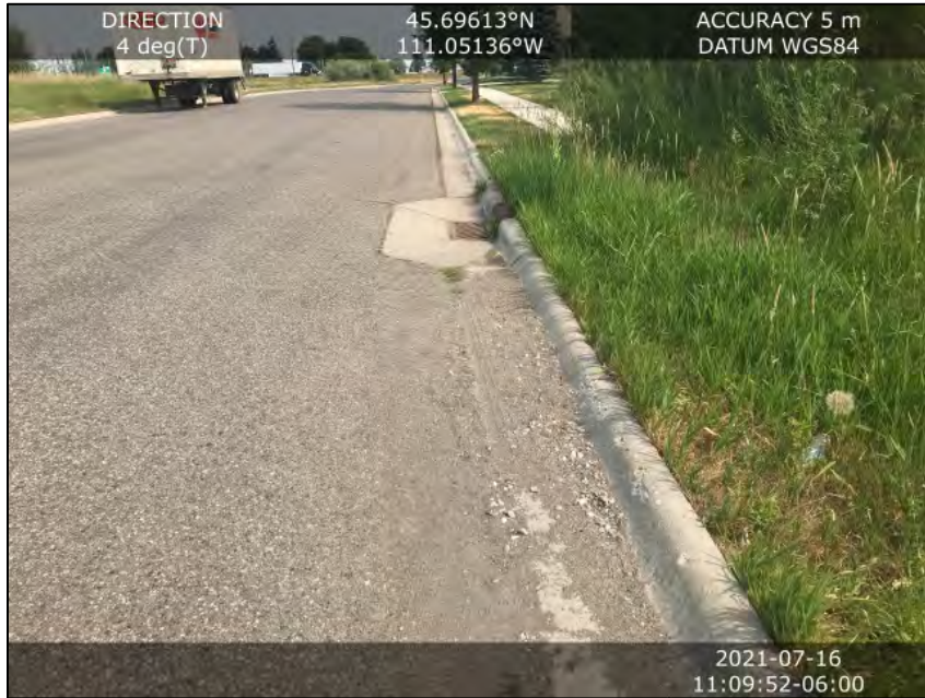
Image 1 Facility overview, detention facility toward right where curb ends (north view).
