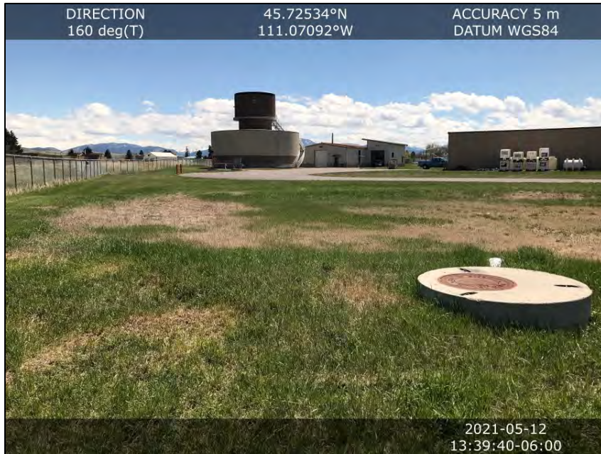
Image 1 Outlet structure and east half of the facility. (south view)
