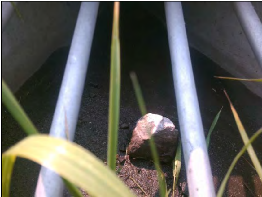
Image 5 Inlet 2 close-up inside trash rack.
