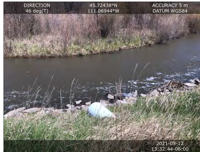
Image 2 Outfall. (north view)
