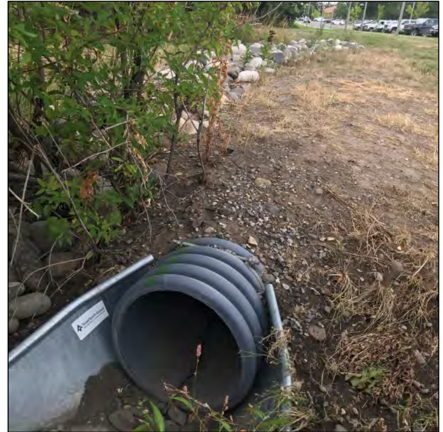
Image 4 Outfall, 18" HDPE (east view).
