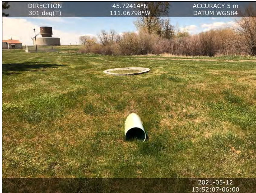
Image 3 West half of facility, outlet and outlet structure. (northwest view)
