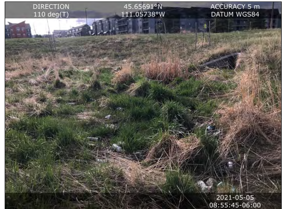
Image 2 Facility inlet with sediment and trash beginning to accumulate. Overall, taking a very small amount of volume. (east view)
