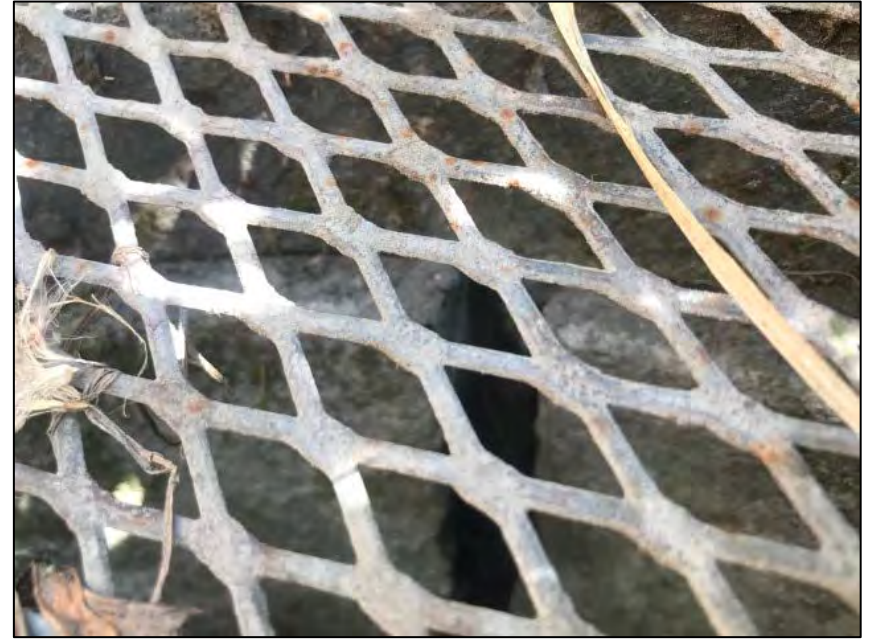
Image 4 Outlet structure; notched weir closeup.
