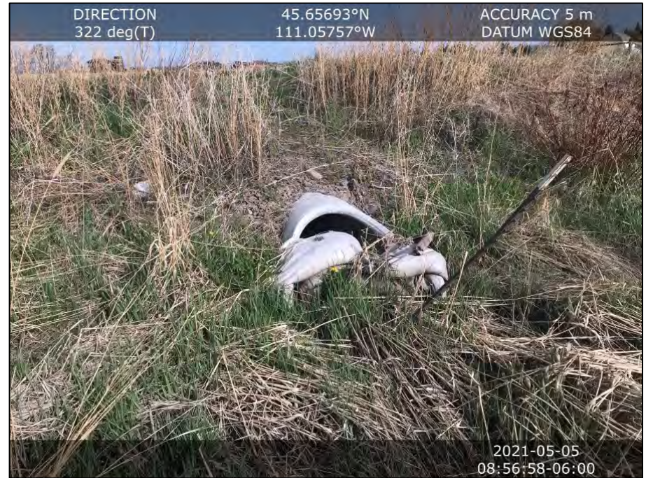
Image 4 Facility outlet to outlet structure. Sand bags are intact but not meant to be permanent. There is one phase of construction still to be completed which leads to this facility. (west view)
