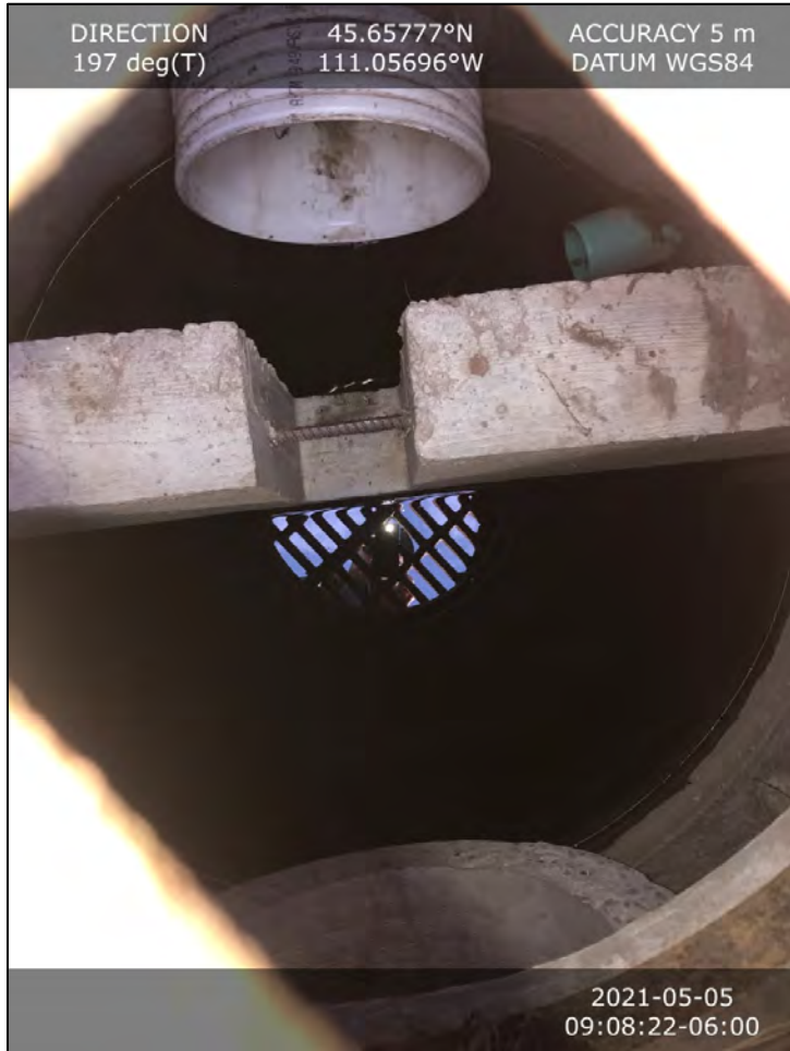
Image 3 Inside the outlet structure.
