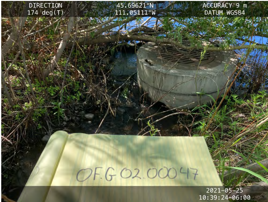
Image 3 Water flowing through facility / around outlet structure
