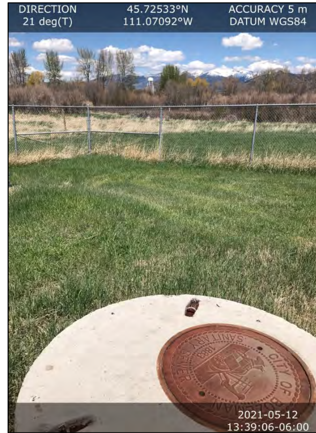
Image 4 Outlet structure. Outfall is inside the fenced area. (north view)
