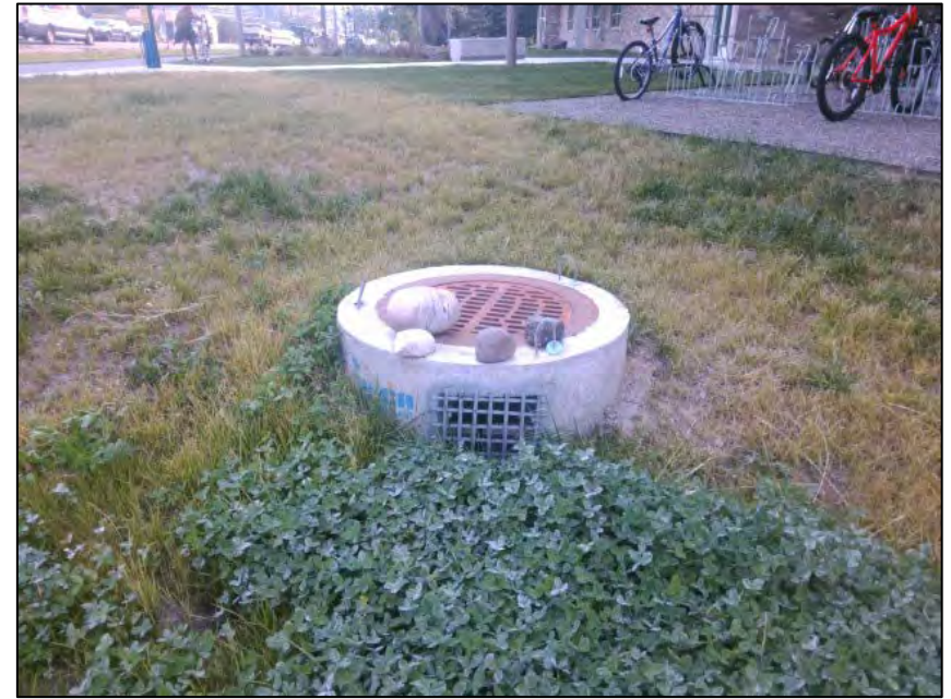
Image 4 Surface outlet structure.
