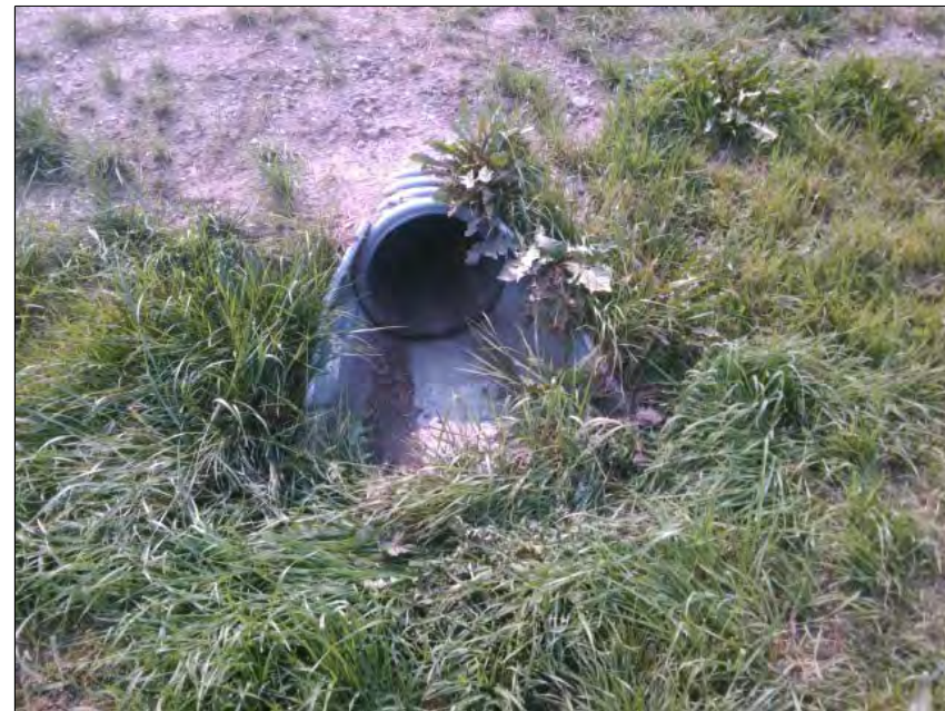
Image 2 Basin inlet from manhole. 15" HDPE (south view).
