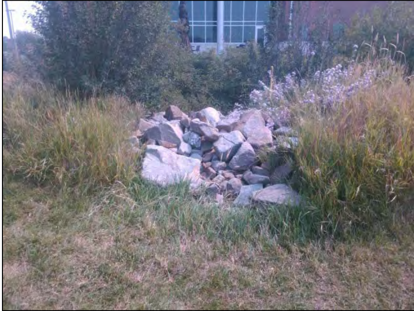
Image 3 Overflow with riprap armoring (east view).
