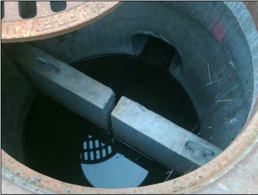
Image 5 Outlet structure weir.
