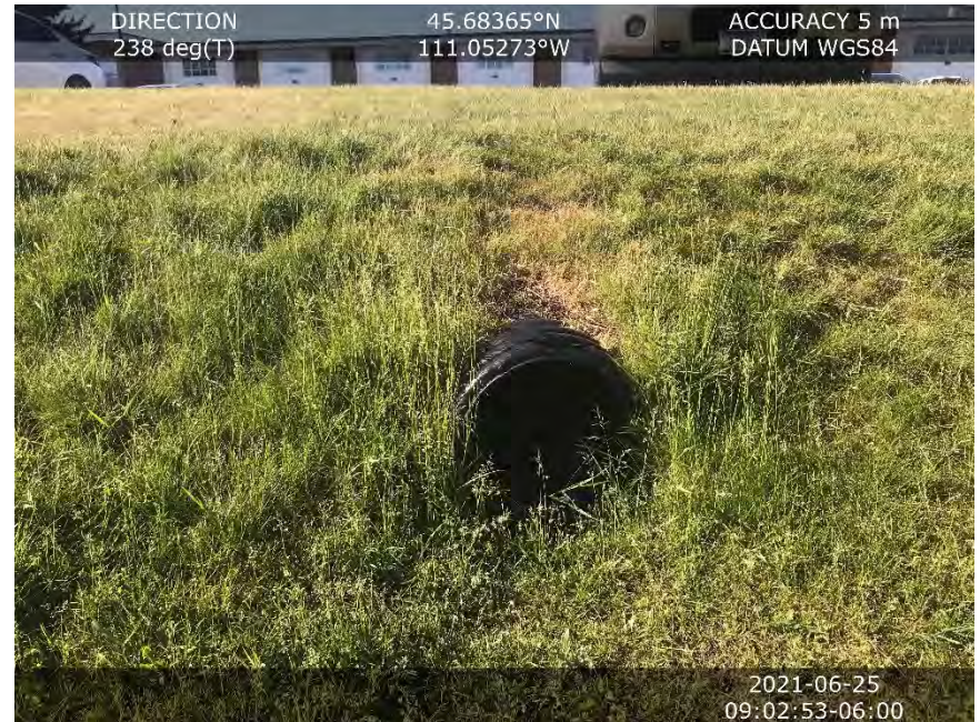
Image 4 Second inlet from south. (south view)
