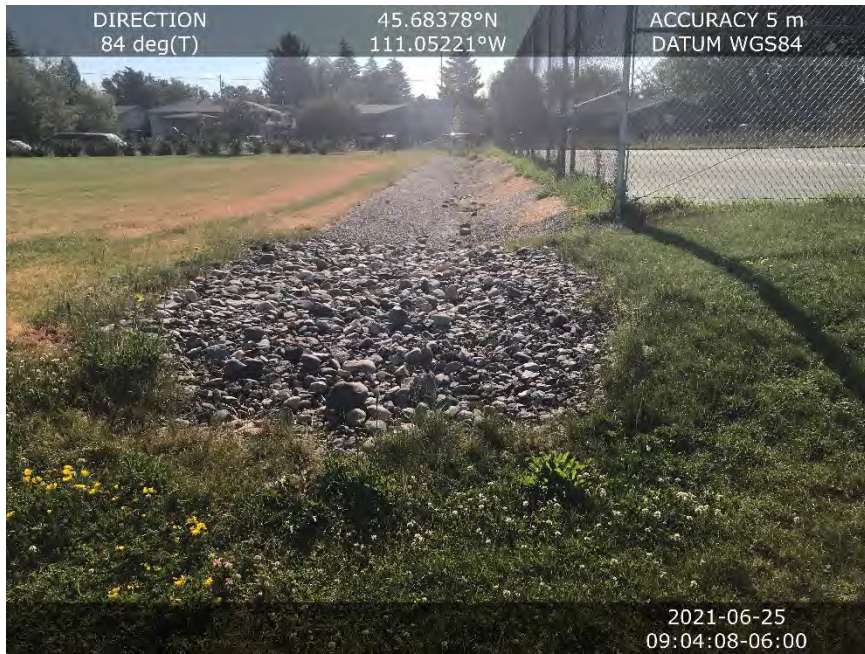
Image 5 Overflow channel of gravel and asphalt leading to Mandeville Creek. (east view)
