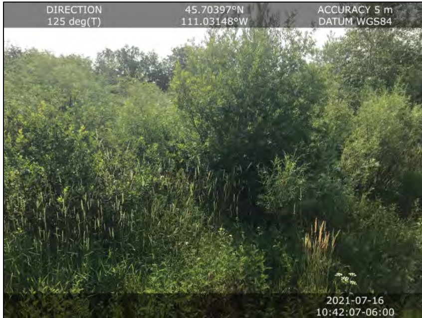
Image 1 Severely overgrown detention basin
