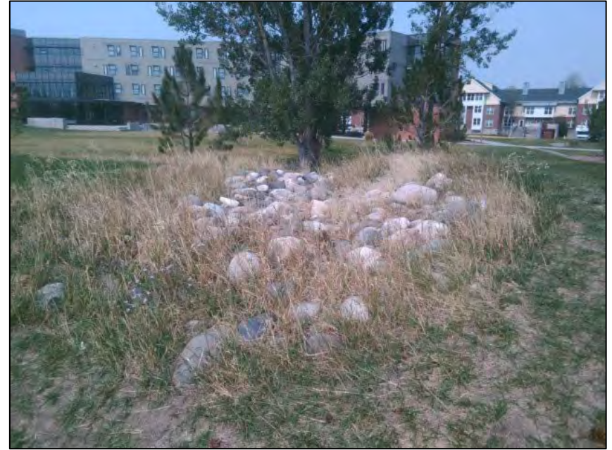
Image 4 Cobble reinforced emergency spillway.
