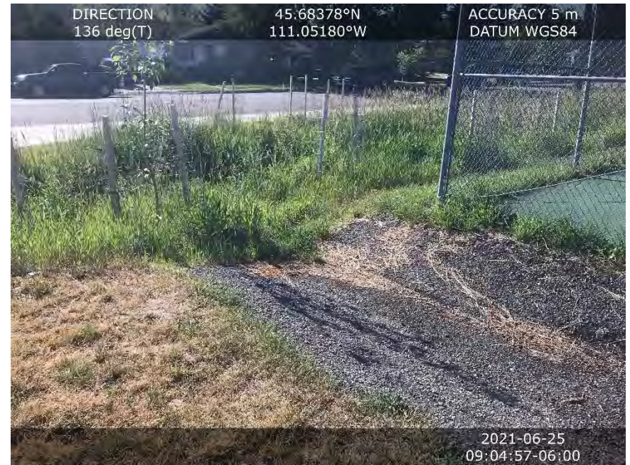
Image 6 Overflow channel and outfall. (southeast view)
