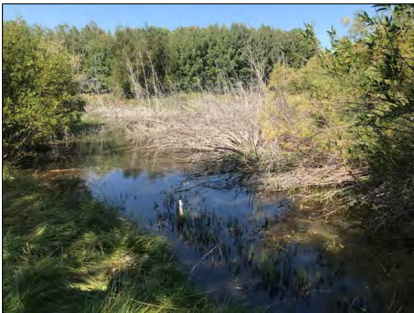
Image 1 Detention pond (west view); standing water, dead and decadent tree and shrub vegetation layer.
