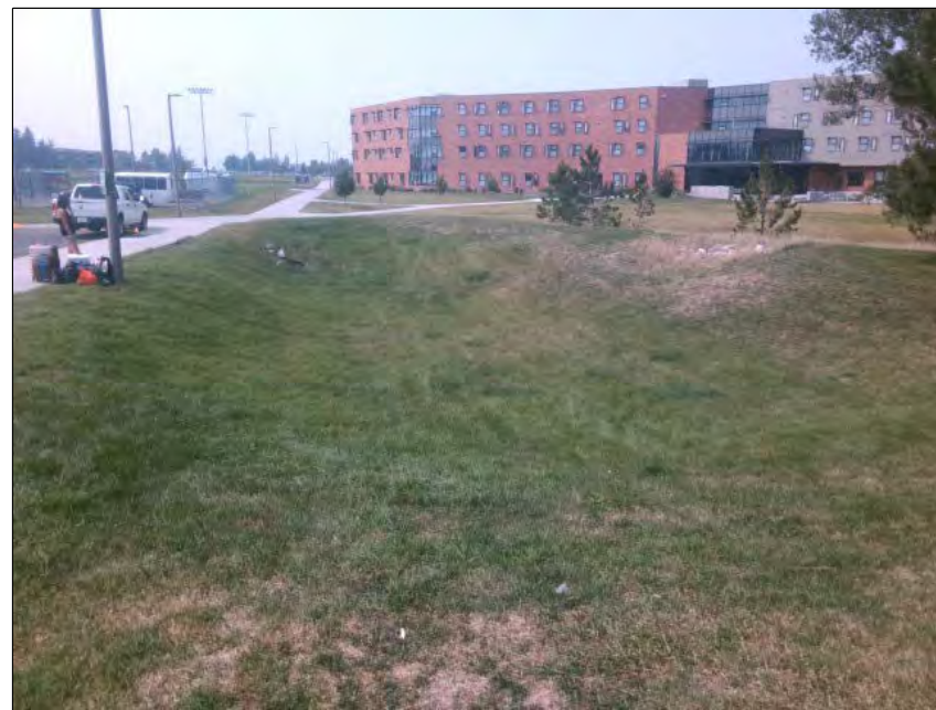
Image 2 Emergency overflow. (West view)
