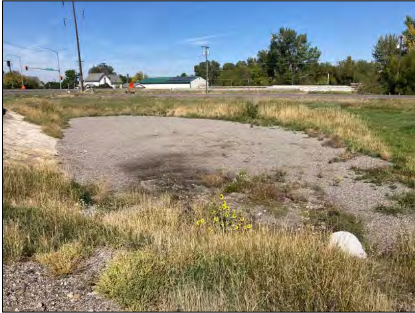
Image 1 Facility overview. Main pond inlet at foreground (white PVC). Note gravel installed on bottom of impoundment (northwest view).
