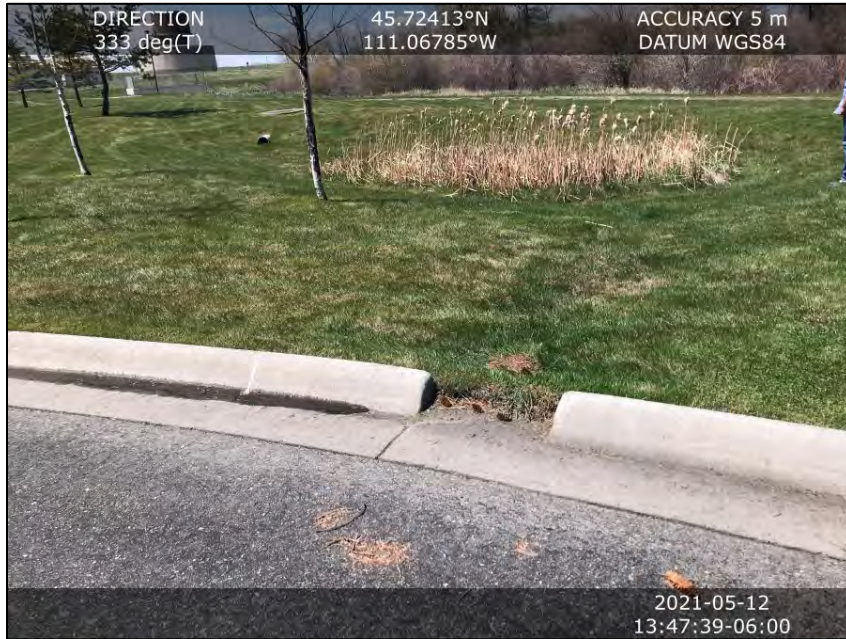
Image 1 Facility overview. Curb cut at foreground has been cleaned out since last year and curblines have been swept. (north view)
