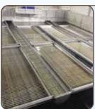
The flocculated suspended particles and chemical settle out in the sedimentation basin. Inclined plate settlers speed up the settling process. The sludge that is formed is pumped to the solids handling processes.
