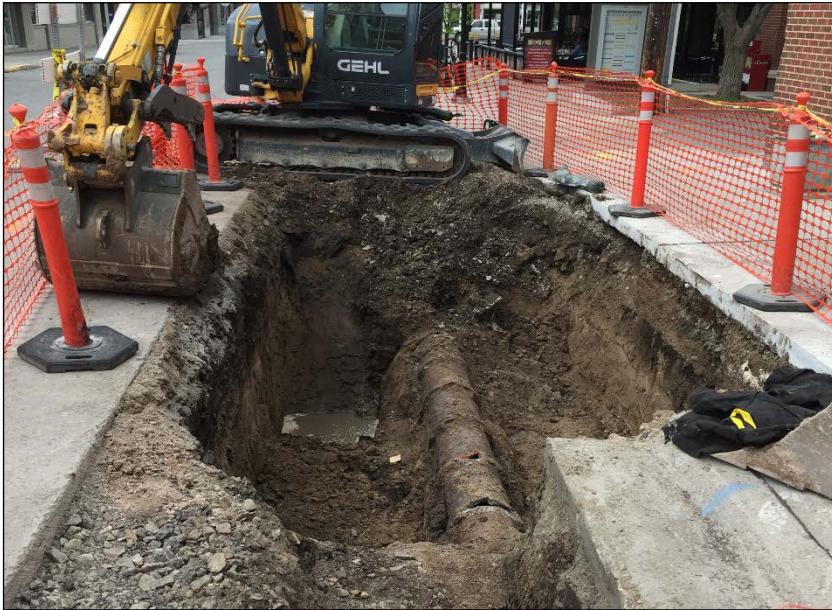
Graphic: Stormwater treatment unit installation
