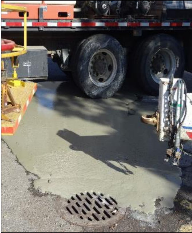
Graphic 4.0.1: Bentonite slurry spill
