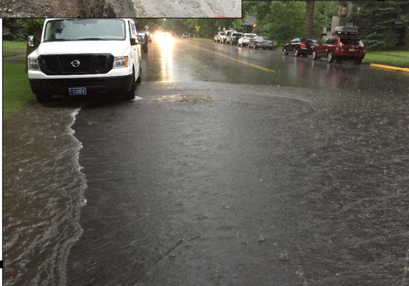
Graphic: Surcharging storm sewer utility structure
