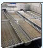
The flocculated suspended particles and chemical settle out in the sedimentation basin. Inclined plate settlers speed up the settling process. The sludge that is formed is pumped to the solids handling processes.
