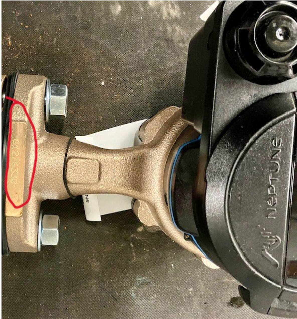
1. 1.5" and larger Mach 10 ultrasonic meter serial number on brass flange
