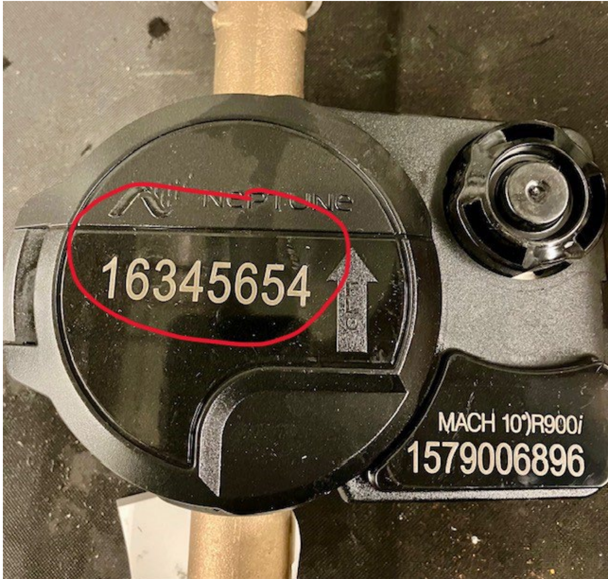
All sizes of Mach 10 ultrasonic meter MIU housing lid with meter serial number
