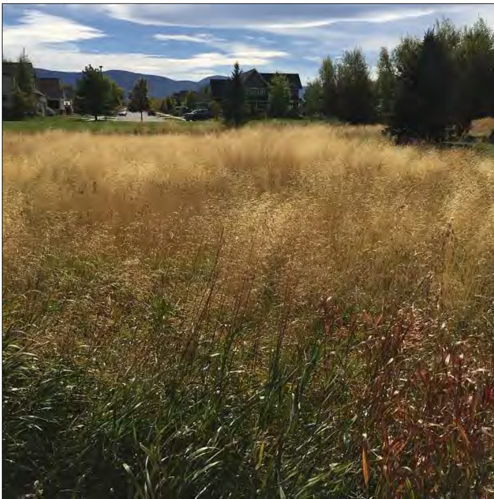
Image 1: Stormwater basin overview displaying overgrown vegetation (south view)
