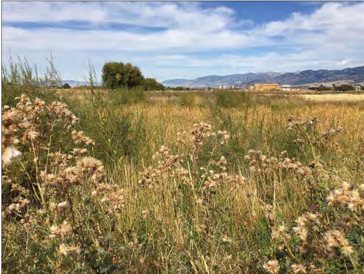
Image 6: Stormwater basin overview showing overgrown vegetation (north view)
