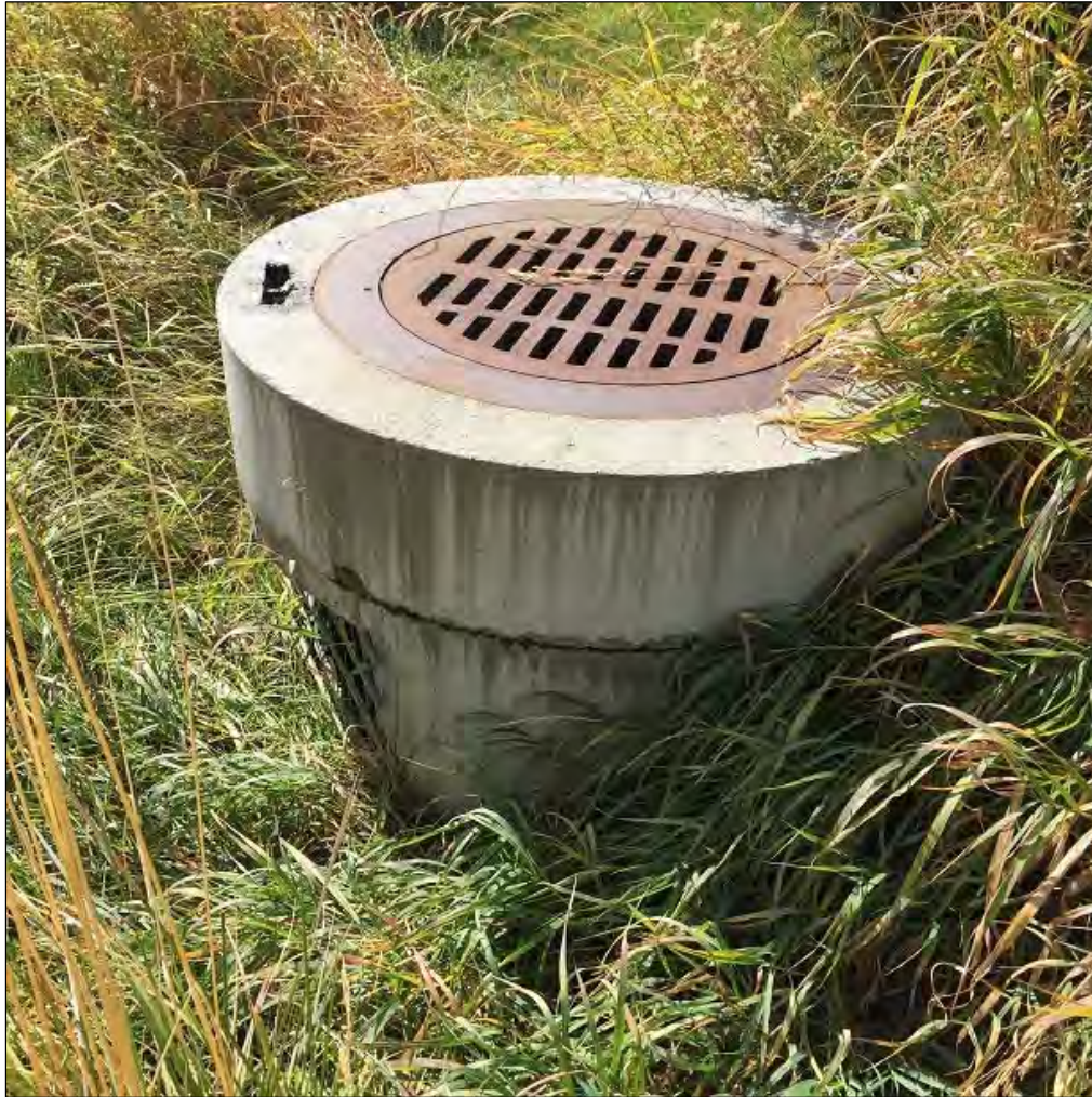
Image 4: Outlet structure overview (south view)
