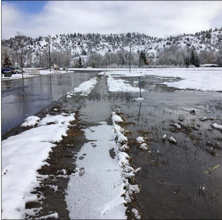
Graphic 1.0.1: Street-flooding resulting from clogged infrastructure
