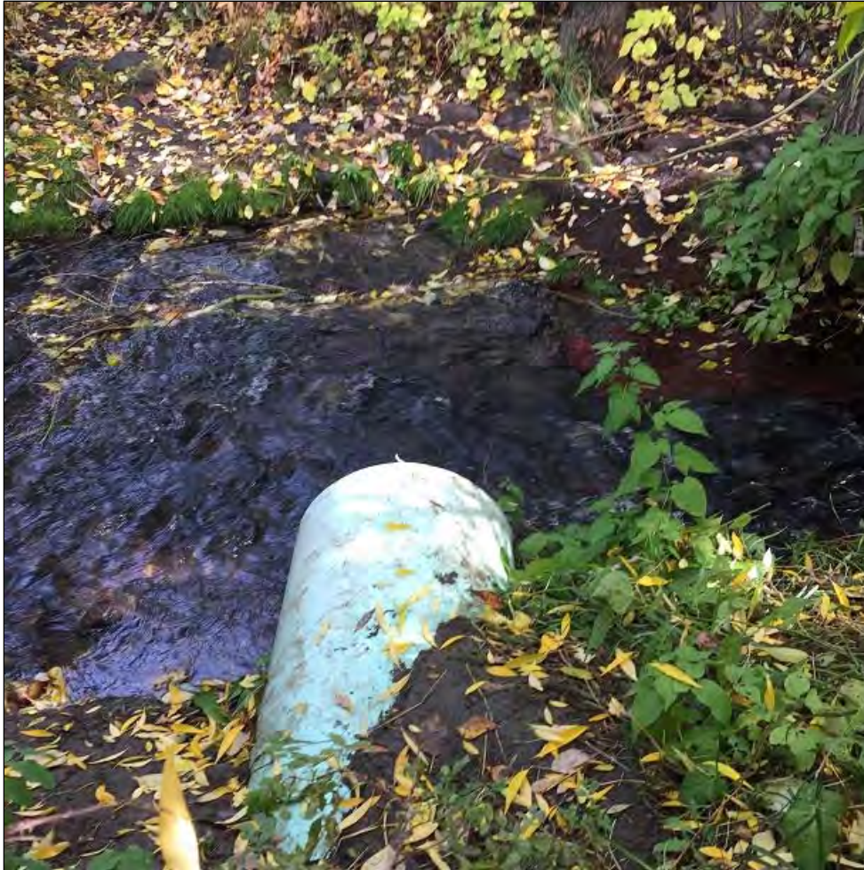
Image 5: Stormwater basin discharge pipe (east view)
