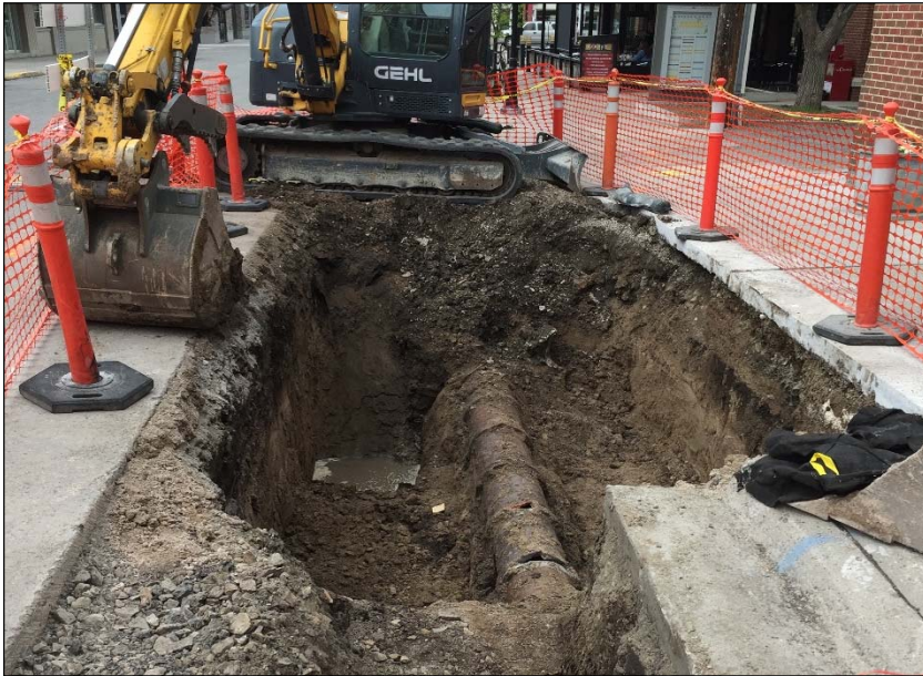
Graphic: Stormwater treatment unit installation
