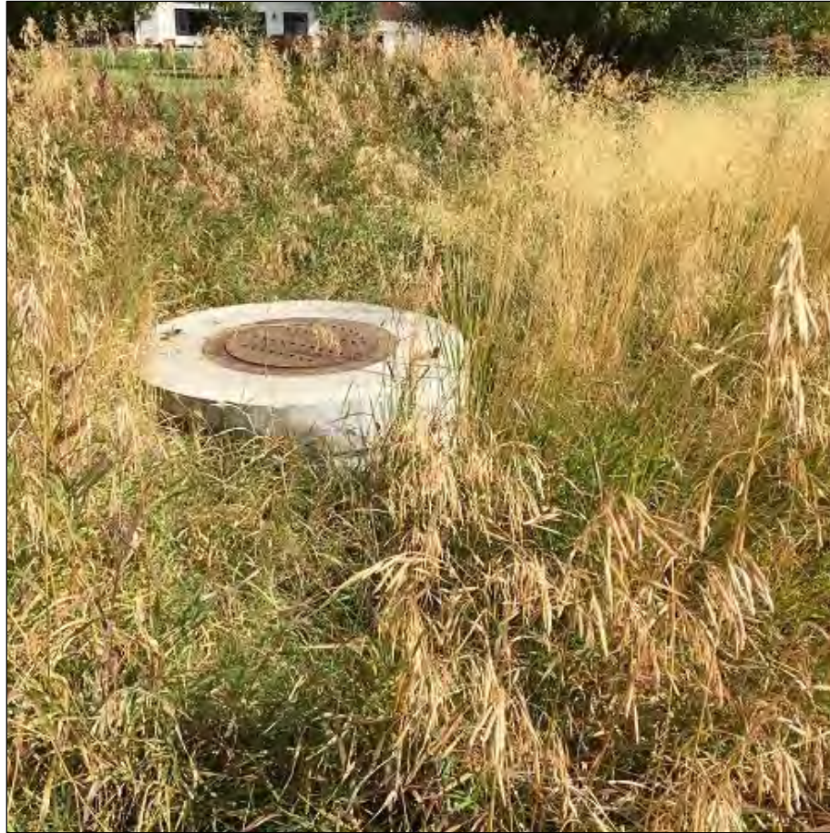
Image 4: Outlet structure overview (north view)
