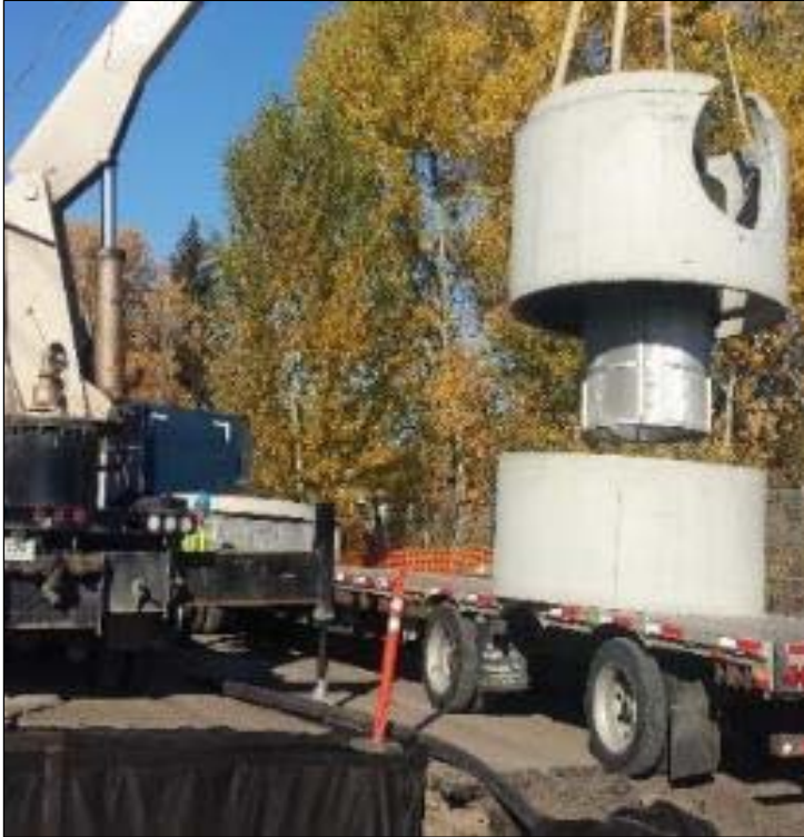
Graphic 2.0.1: Stormwater treatment unit installation
