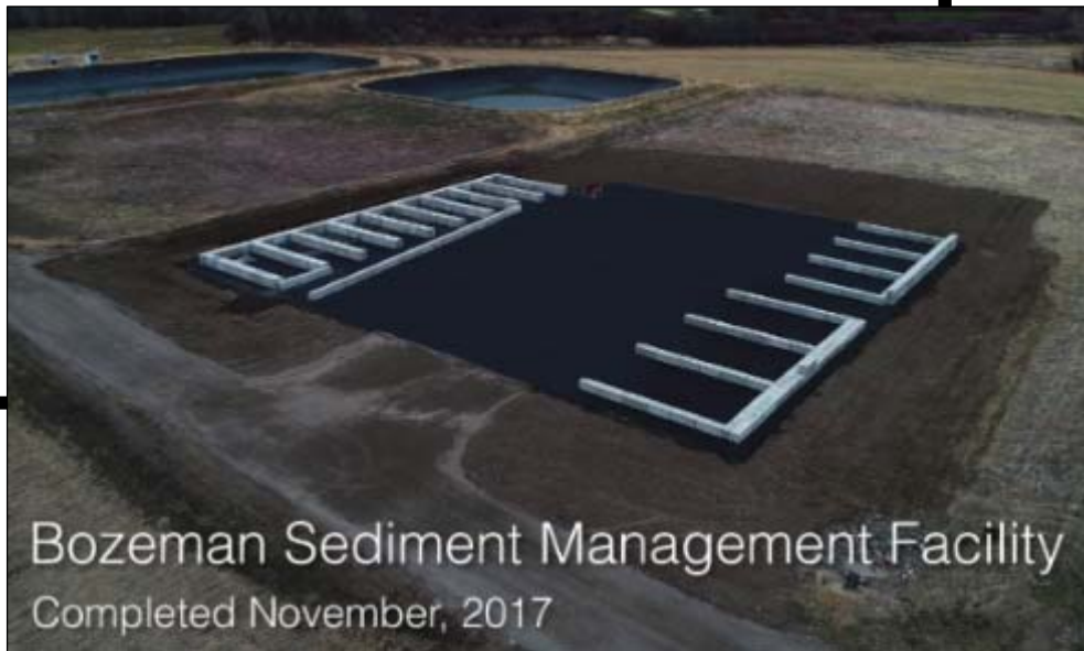
Graphic 7.0.2: Sediment management facility
