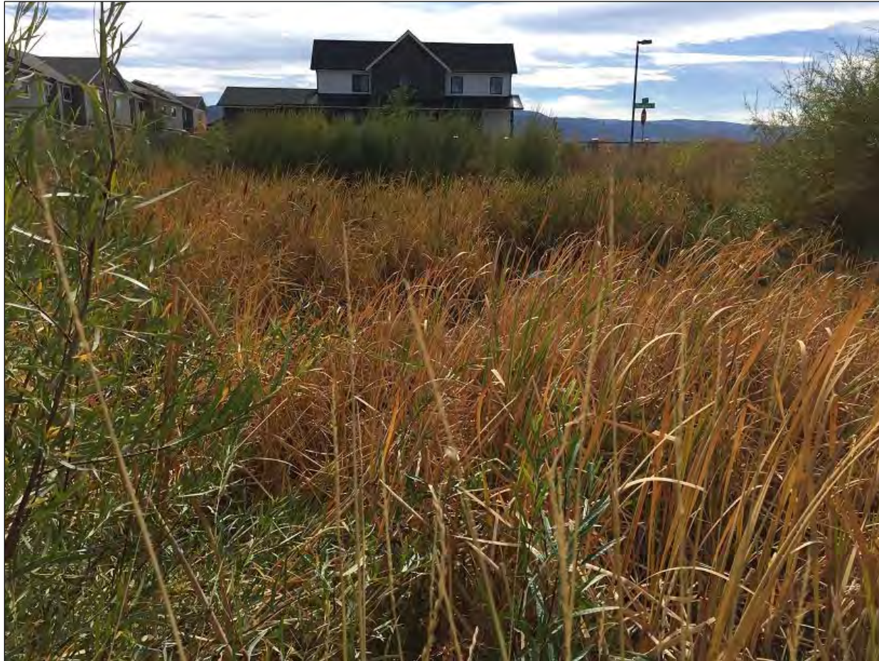
Image 2: Stormwater basin overview displaying overgrown vegetation (south view)
