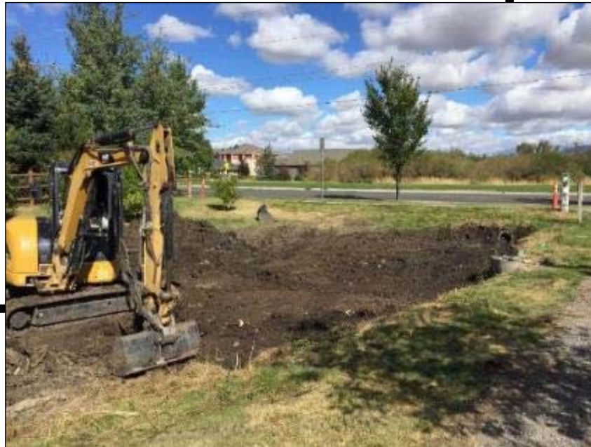
Graphic 6.0.2: Dredged stormwater basin
