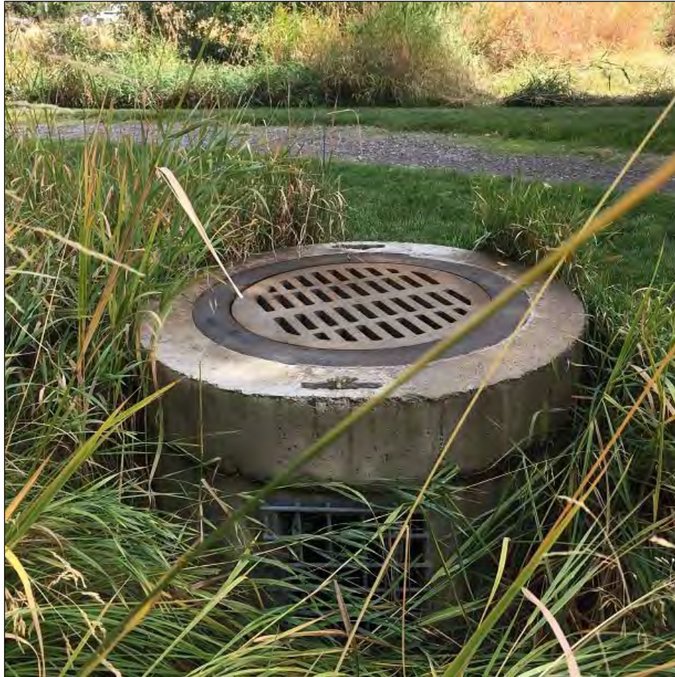
Image 4: Outlet structure overview (east view)
