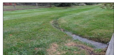
Image 3 - Erosion causing channelized flow
