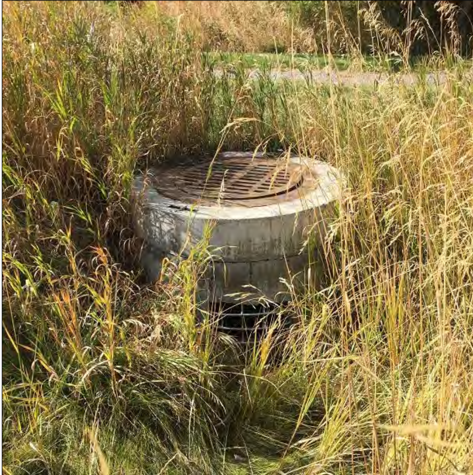
Image 4: Outlet structure overview (west view)
