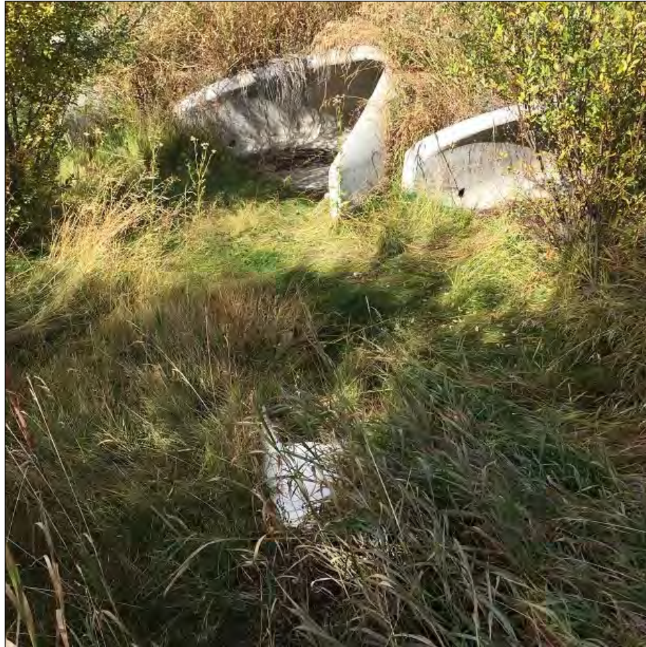
Image 5: Stormwater basin discharge pipe (north view)
