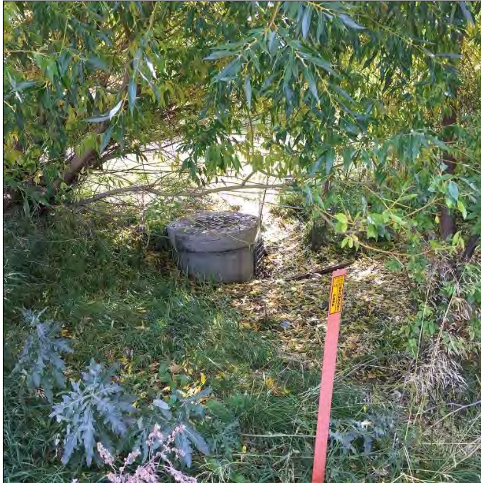
Image 4: Outlet structure overview (east view)
