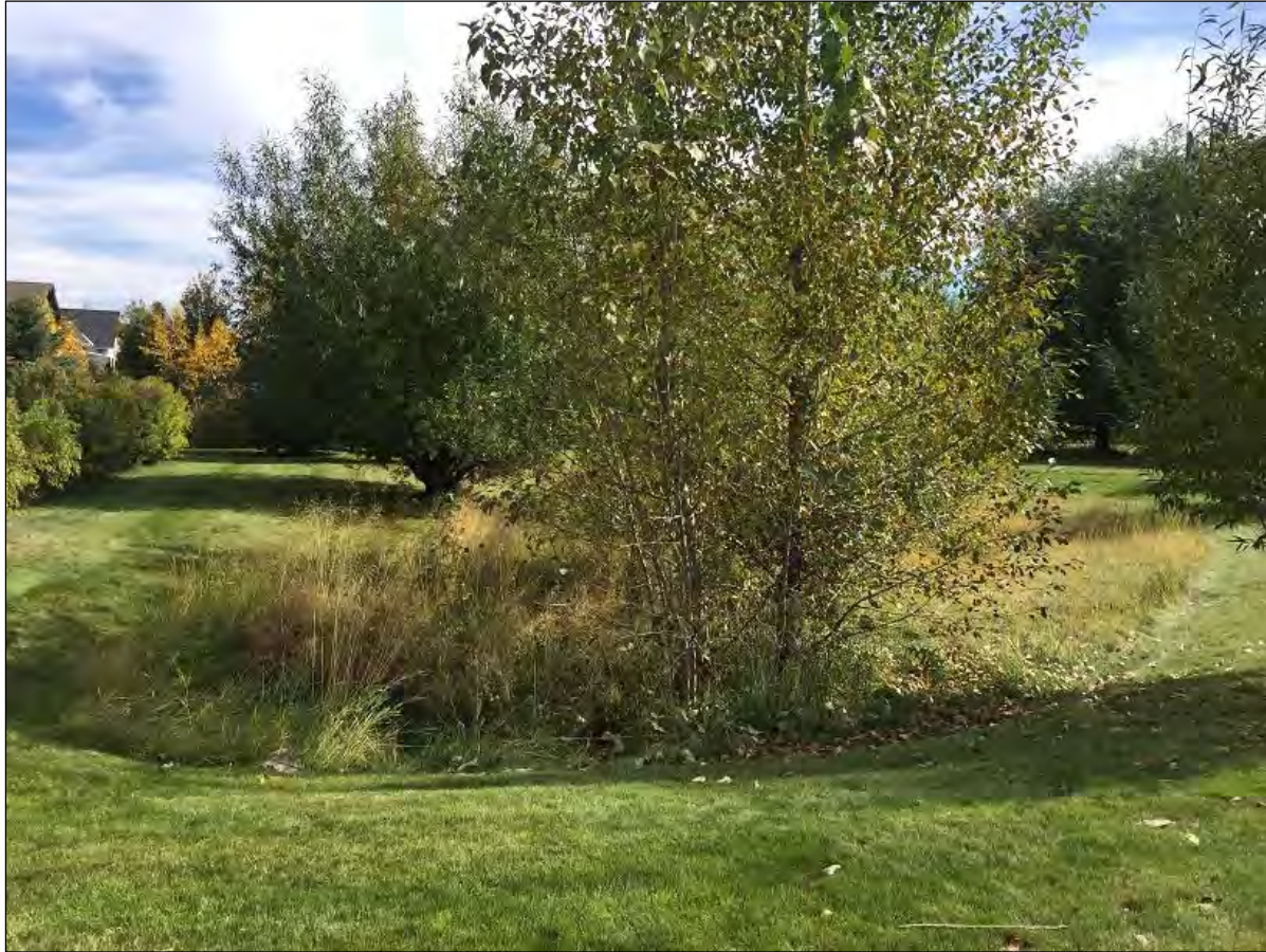
Image 1: Stormwater basin overview displaying overgrown vegetation (east view)
