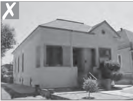
If stucco covers original siding, then its removal is encouraged.
