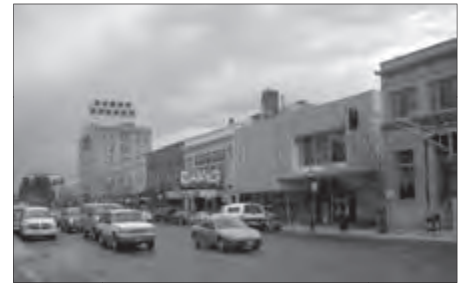
Use building forms similar to those found traditionally. Rectangular shapes are typical and are encouraged.
