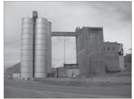
The Historic Story Mill complex uses many different materials such as wood, metal, and stone.
