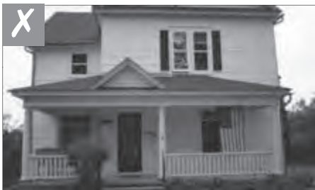
Consider removing later covering materials that have not achieved historic significance. Compare the left photo with the photo on the right, after the synthetic siding was removed. Note how the lap dimensions on the original siding are much smaller.
