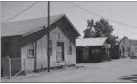
Build upon the “industrial style” architecture that exists along the Story Mill Historic District.
