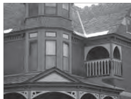
Protect and maintain significant stylistic features, such as these porches, roof lines and window details.
