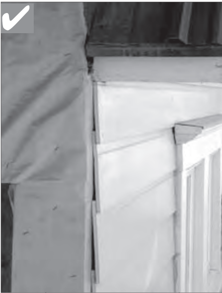
The use of hardiplank horizontal lap siding is appropriate in most residential neighborhoods outside of the historic district.
