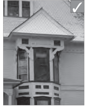
Protect and maintain significant stylistic features, such as this window detail.
