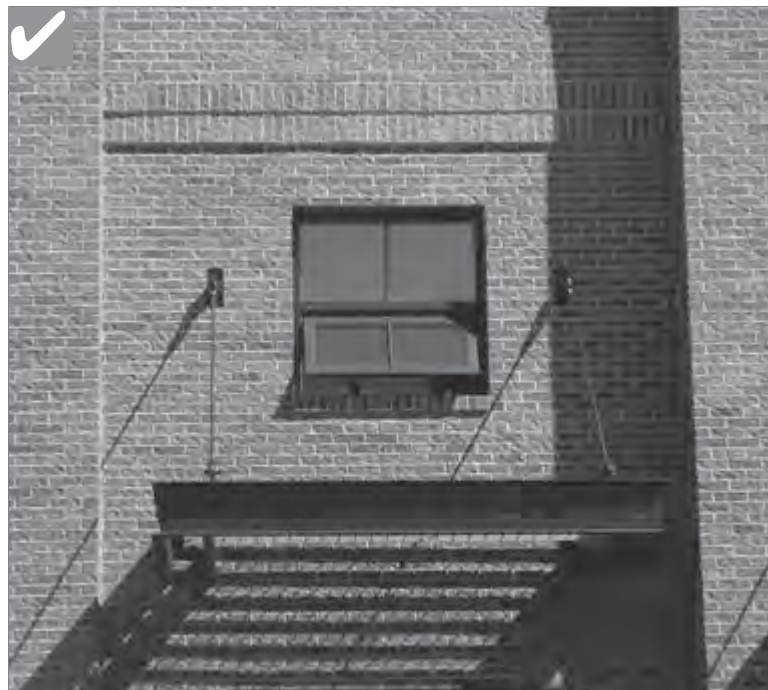
The use of masonry that appears similar in character to that seen historically is appropriate.
