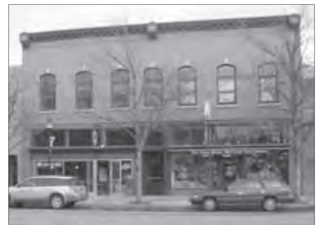
Traditional Main Street building facade.
