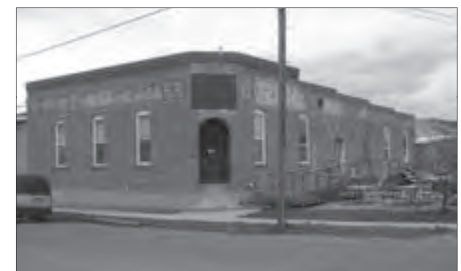
This building reflects the district's industrial character. Brick was the predominant material on the brewery building.
