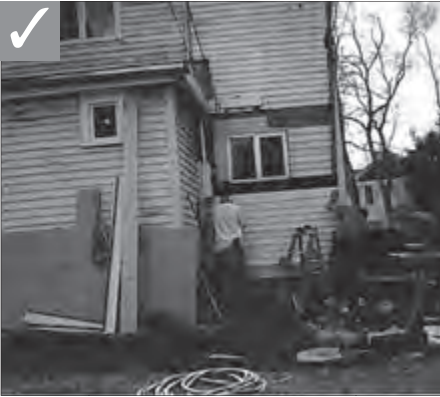
Repair wood features by patching or piecing-in new wood elements that match the original.
