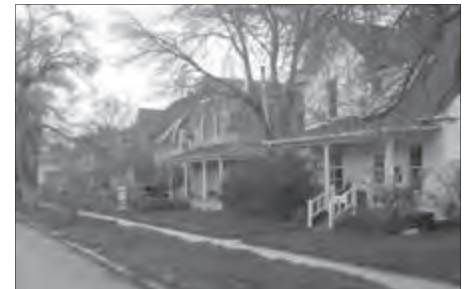
Building setbacks are uniform on this block in the district, therefore new buildings should conform to this alignment.
