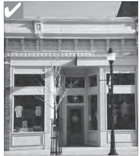
The first floor of a commercial building should be primarily transparent.
