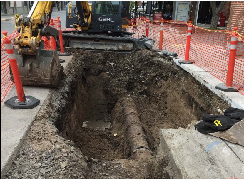
Graphic: Stormwater treatment unit installation
