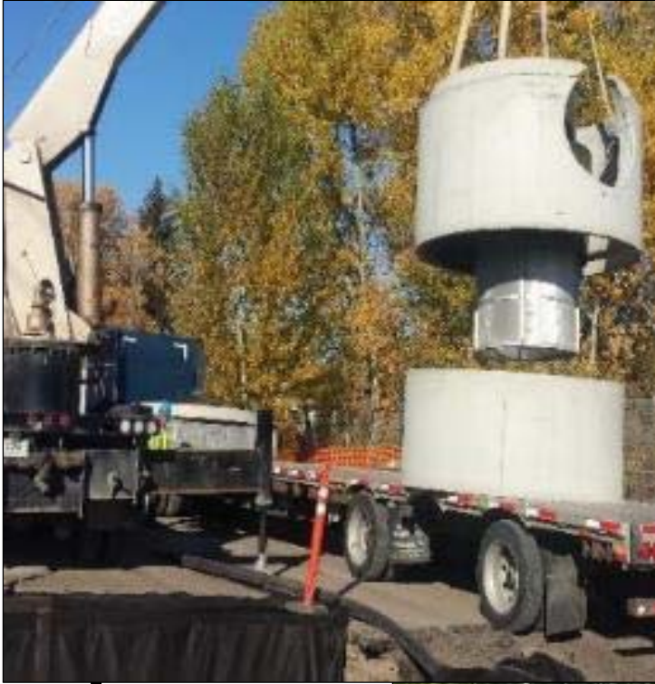
Graphic 2.0.1: Stormwater treatment unit installation
